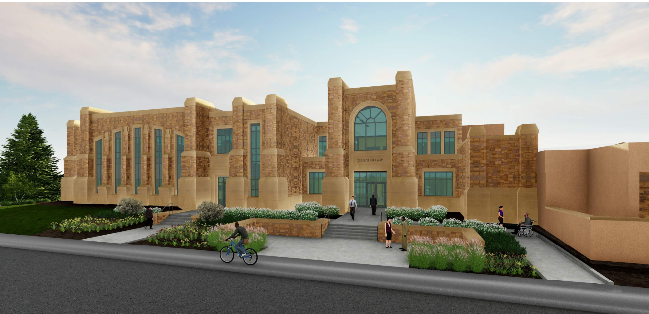
View - New Main Entry
