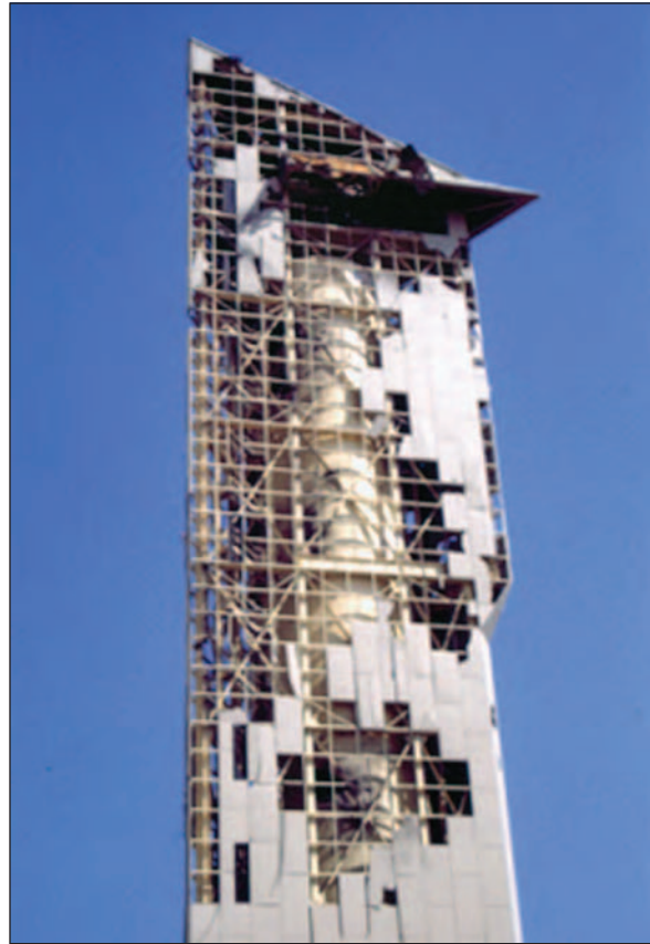
Photo courtesy of Capt Charles G. Grow The water tower in southern al-Khafji was heavily damaged during the battle. It was a favorite target for both Iraqi and Saudi troops and was strafed at least once by U.S. Marine Cobra helicopters.
