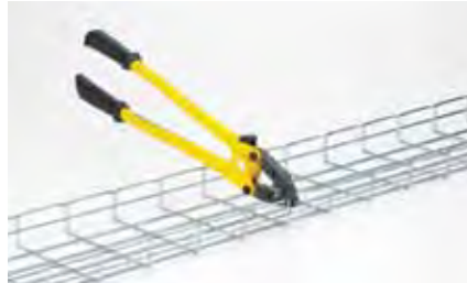
2 Turn tray to the side with open side facing you. Repeat step 1 to cut wire.
