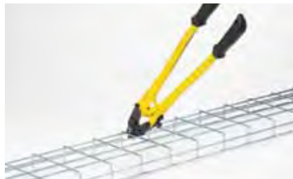
5 Finish cutting by moving to other side of tray to cut remaining wires,
