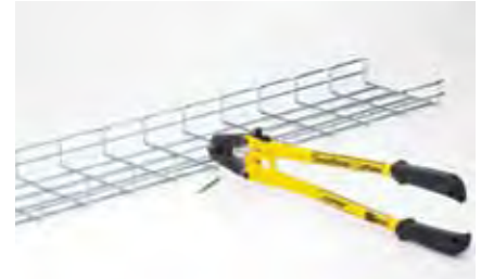
3 Finish cutting all side wires.
