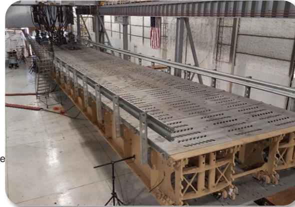
Long semi-permanent tactical bridge
