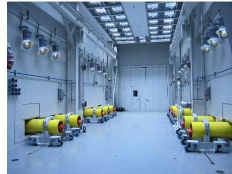
PEVEL - Test Cell Interior
