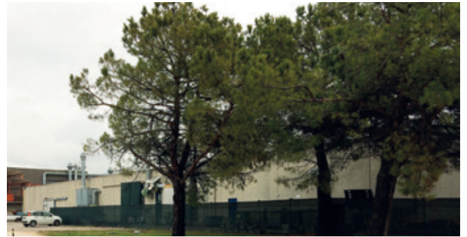
UFLEX - Factory in Tregnago
