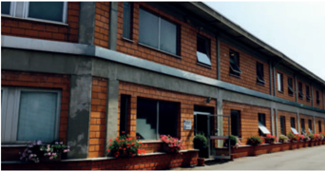
UFLEX & ULTRAFLEX - Headquarter in Busalla
