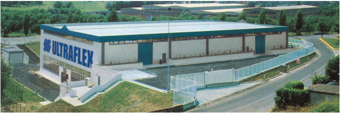
ULTRAFLEX - Factory in Casella
