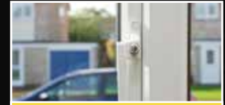
Double Glazing Lock Repairs
