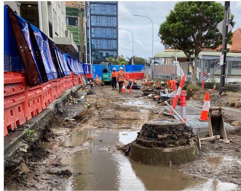
Photo 10 – Roadworks on Little Eveleigh Street. Jersey barriers and noise blankets installed to enclose the site and mitigate noise
