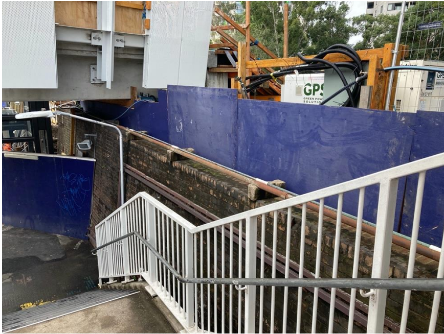
Photo 6 – Protection installed on Platform 10 heritage wall.
