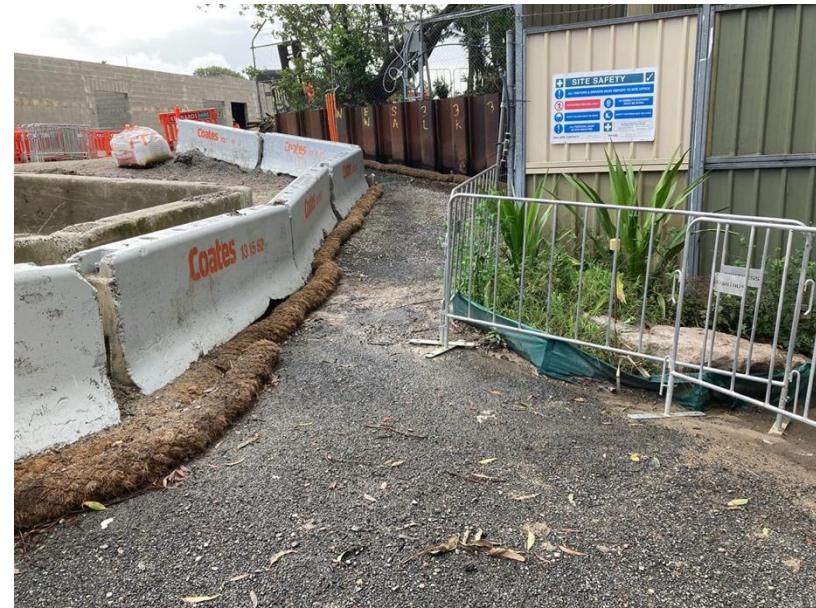
Photo 3 – Erosion and sediment controls on Marian Street compound.
