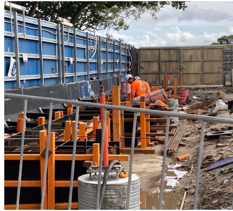
Photo 12 – Construction of footings for bollards on Marian Street.
