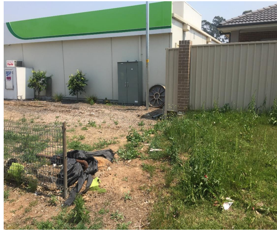
Photo 2 showing metal pipe in the vicinity of the service station, possible underground storage tank in the vicinity of pavement.
