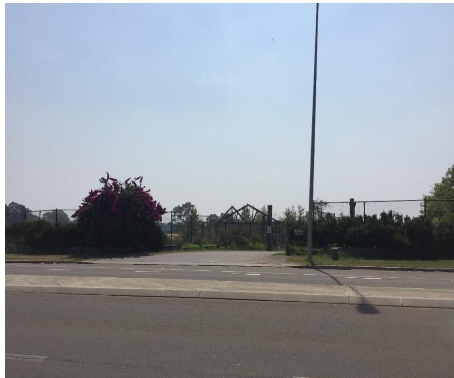
Photo 4 looking southeast from Garfield Road East, note the building in disrepair in the background.
