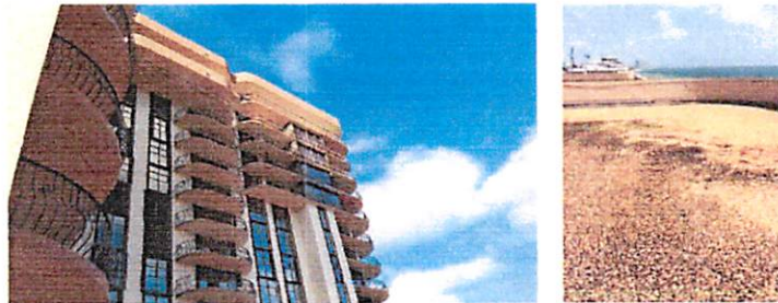
Figure H: No suspension hooks at the underside of the balconies and on the roof.
