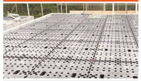
Swale deck safety decking / crash deck, 2m high x 1.2m² panels
