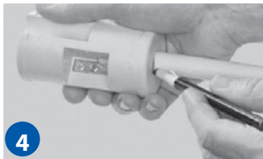
1 Cut the tubing so that the end is square.
