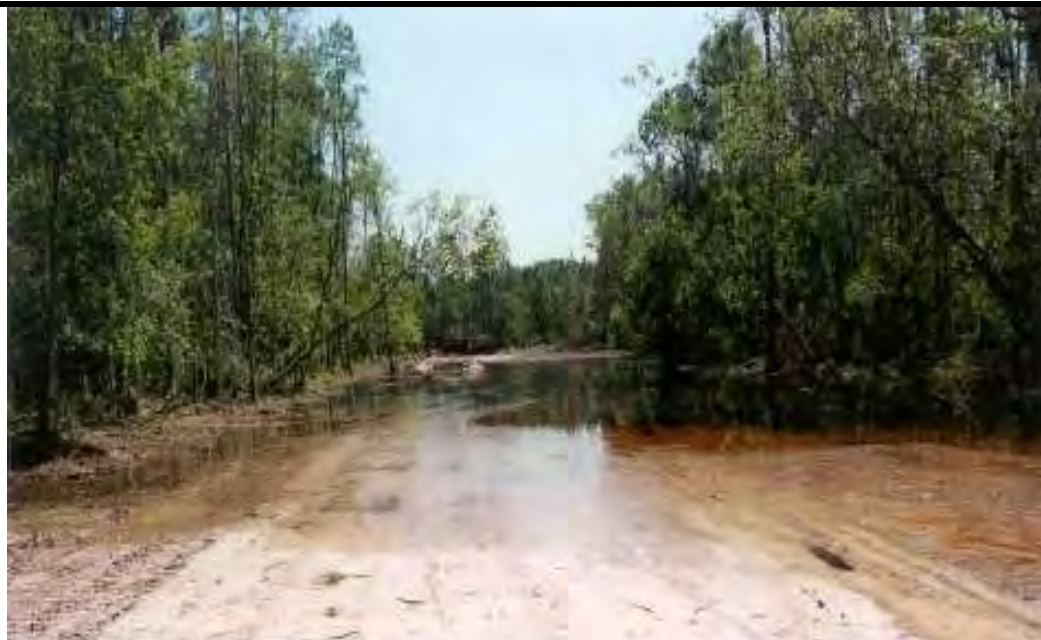
Spring, 2001 – view of the 1.3 mile east-west ditch prior to construction. The associated tram road fill material is located adjacent to the road (right). The substantial ditch dewatered the adjacent wetlands and the tram road diverted historic wetland drainage flow patterns.
