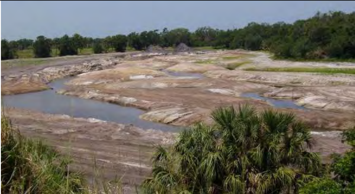
During Construction (2005) – view from atop observation mound, looking west over upland field graded to construct braided tidal channels and marsh zones.
