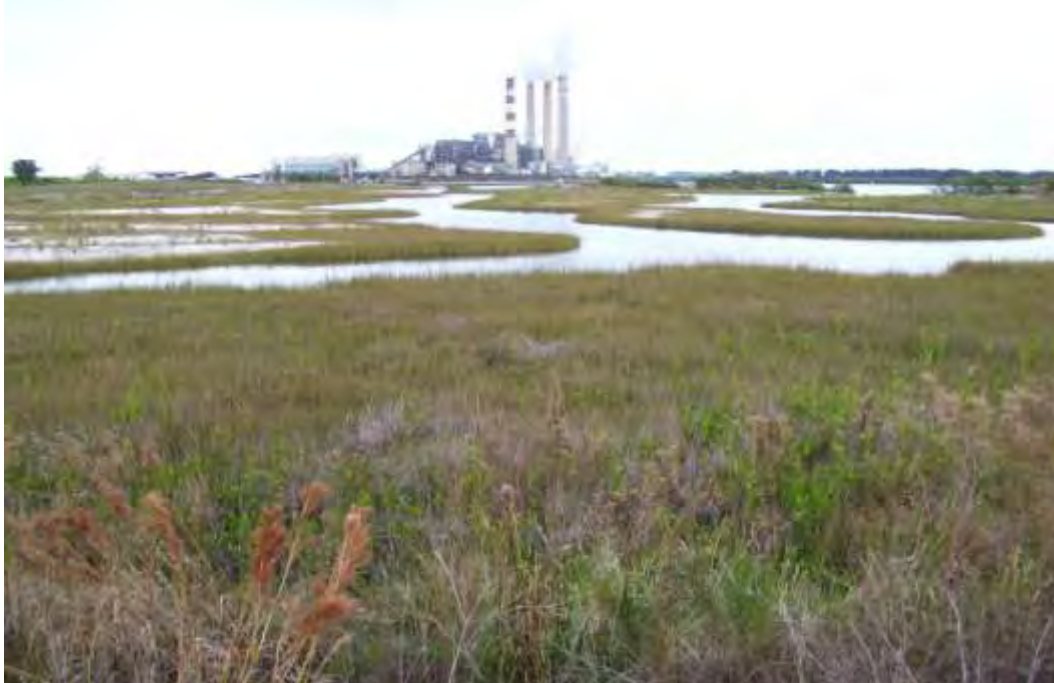
Current Constructed Conditions (2009) - view from the western edge of the project looking north over the created salt-marsh & inter-tidal channel habitats (TECO Big Bend Power Plant in background). The low salt-marsh habitat provides the designated FDOT mitigation, with dominate coverage provided by smooth cordgrass with naturally recruited mangroves. The high salt-marsh has dominant coverage of salt-grass, seashore paspalum, marsh-hay cordgrass; as well as areas of rare saltern habitat (upper left).
