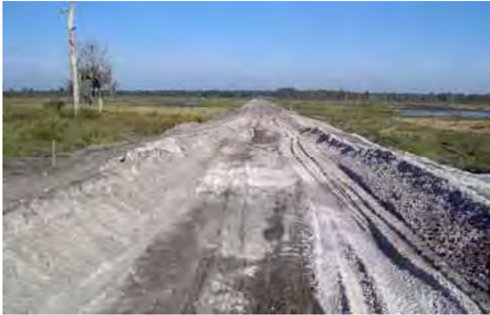
Standing on the southern end of the Center Road looking north. Fill material was used to elevate the remnant road (3,050 ft. long), and culverts installed to restore west-east sheet flow hydrology through the restored and enhanced wetland habitat.
