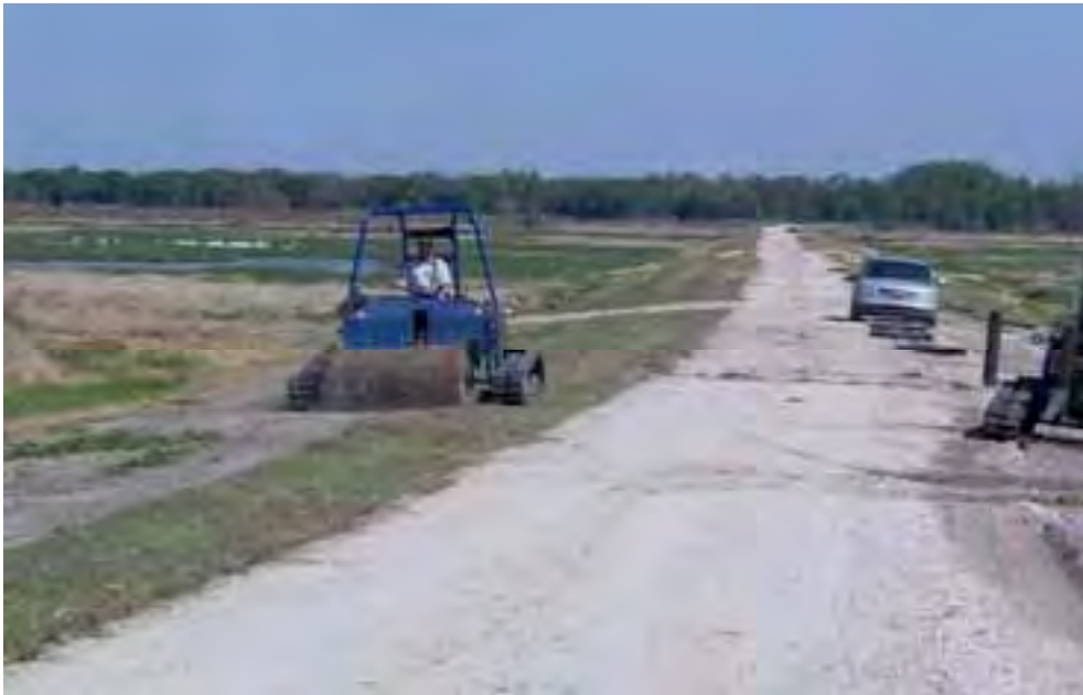
Final construction of the Center Road and sod being installed to stabilize the slopes. Water starting to pool upstream and attracting white pelicans and wading birds (left).
