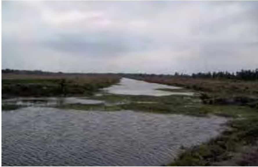
View from Center Road, looking west at the Banana Creek Canal just prior to backfilling with the adjacent spoil material.
