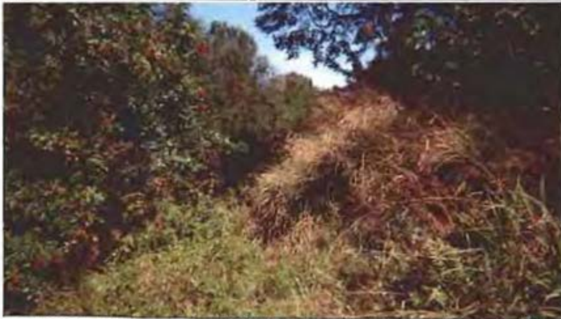
Forested Wetland Enhancement (FWE 1) – One of the large north-south ditches that collects surface water from the uplands and directly discharges to the channelized creek north of property boundary. Spoil material (right) is 15-20 ft. wide and 5-6 ft. high, covered with paragrass and various sedges. This material will be backfilled into the ditch to restore grade, seeded, and planted with shrubs and trees. Additional enhancement will include eradication of Brazilian pepper (left) that has encroached into this wetland.
