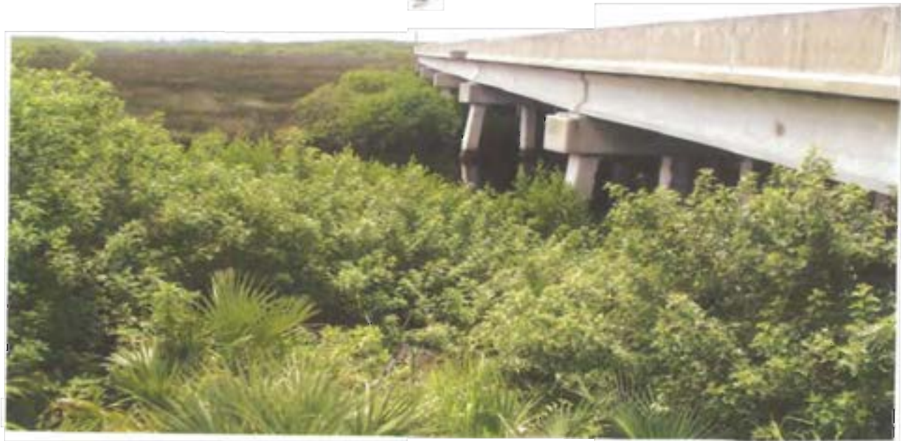
Site A – Pre-Construction (2001) – view from the northern bridge embankment area, looking south over the tidal branch. Brazilian pepper along the embankment (foreground) with mangroves and black rush south of the open water and adjacent to the bridge.
