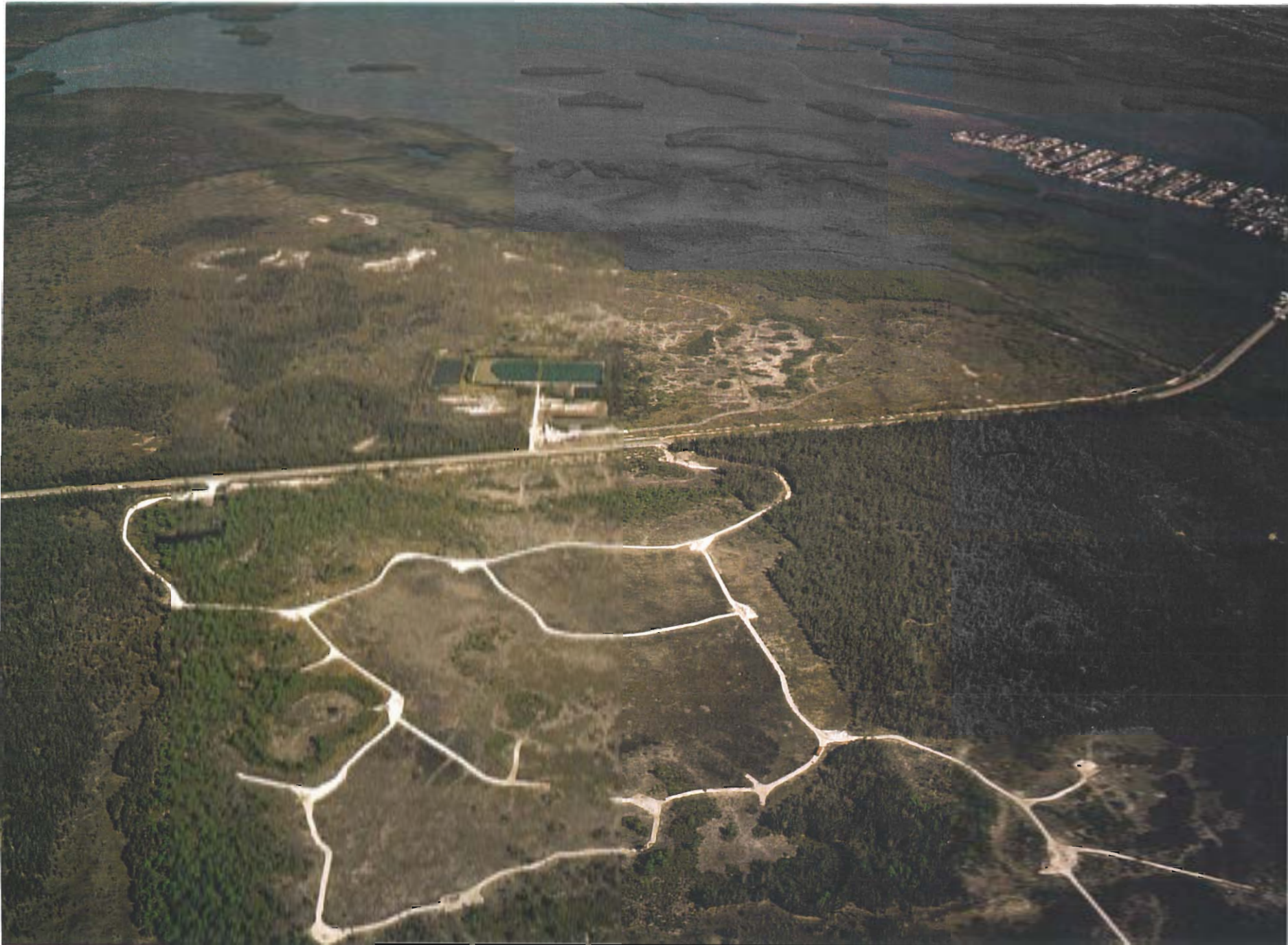
FEBRUARY 2000 - EXOTIC VEGETATION REMOVAL AND HYDROLOGIC RESTORATION OF LITTLE PINE ISLAND COMPLETED IN PHASES I, II, AND V. TEMPORARY ROADS REMOVED FROM PHASES I AND II.
