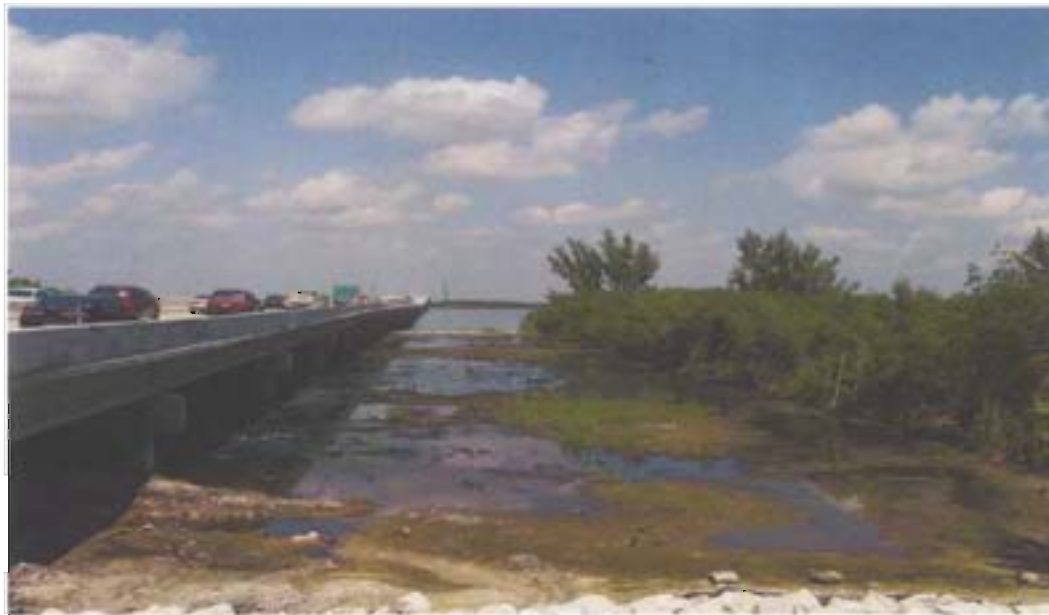
Site C – Post-Construction (Sept. 2003) – the new northbound bridge has been constructed and old bridge removed, exposing bare soil that was under the bridge. The area was planted with white mangrove, black rush and saltmarsh bulrush.
