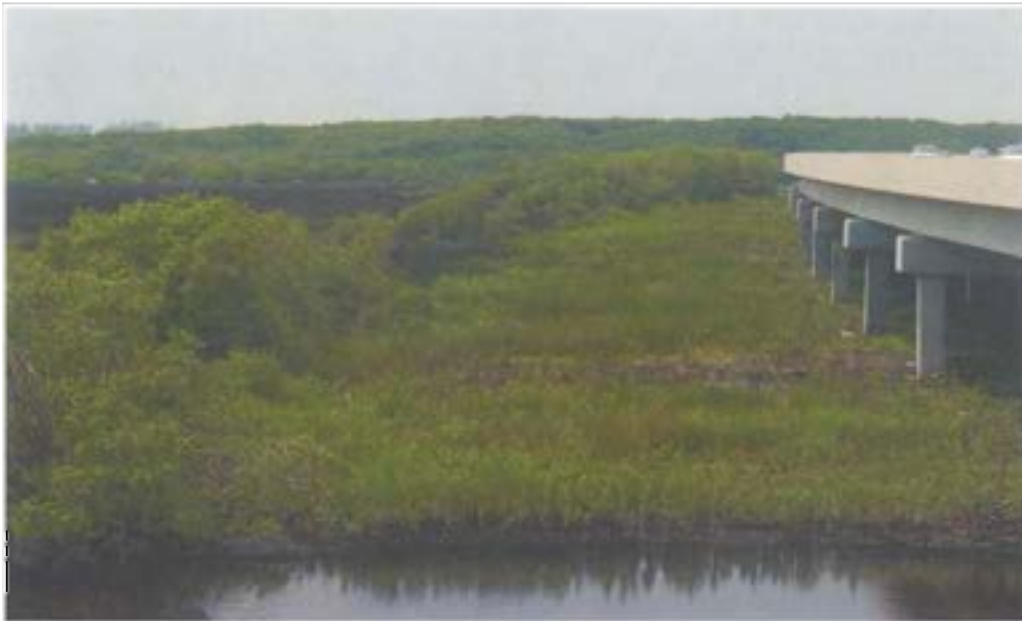
Site A (July, 2004) – planted stock and natural recruitment of desired vegetation provides extensive ground coverage. Herbicide maintenance to eradicate exotics conducted quarterly in 2004 and 2005.
