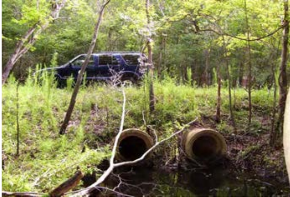
Downstream end of two culverts that discharge water into a creek channel. The culverts will be removed and replaced with rip-rap rubble that will allow gradual seepage into the channel; extending the hydroperiod and attenuation of surface water in the wetland portion on the upstream side of the berm.
