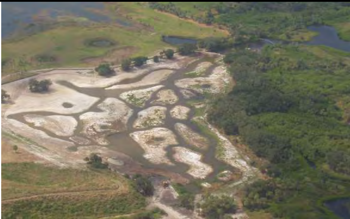
During Construction (2005) – view from atop observation mound, looking west over upland field graded to construct braided tidal channels and marsh zones.
