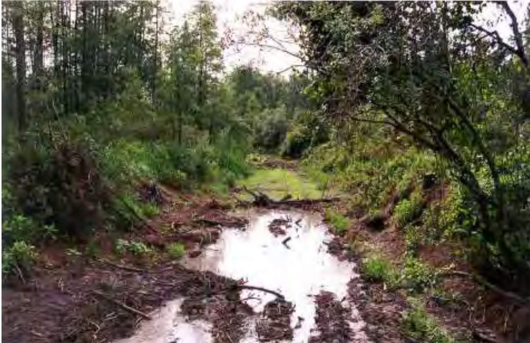
Spring, 2001 – view of the 1.3 mile east-west ditch prior to construction. The associated tram road fill material is located adjacent to the road (right). The substantial ditch dewatered the adjacent wetlands and the tram road diverted historic wetland drainage flow patterns.
