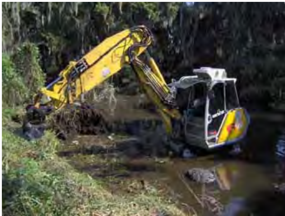
A Menzi unit was utilized in areas where traditional equipment could not access through water, such as this breaching of the rim spoil material to provide hydraulic connectivity to the preserved portion of the Banana Creek Canal.
