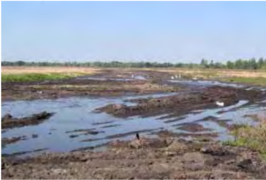
Same view of the Banana Creek Canal a week later, just after filling and prior to planting with herbs such as pickerelweed and arrowhead.
