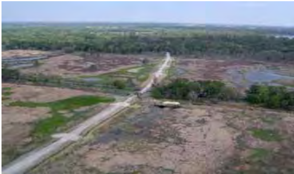
The 2,000 ft. long East Road just after construction. As with the Center Road, the restored sheet flow is evenly distributed by a series of culverts, as well as "saddle" swales installed at lower road elevations to allow overflow during periodic flood events.
