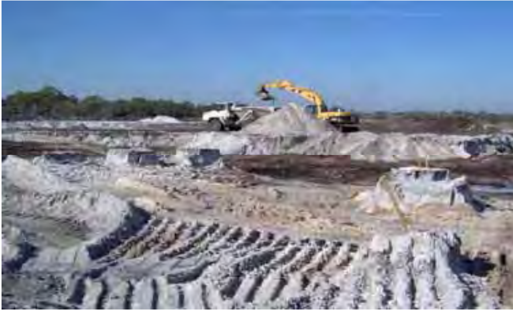
View of the southwest Gator Pond during earthwork activities. Dredging material used to stabilize the Center and Eastern Access Road berms.
