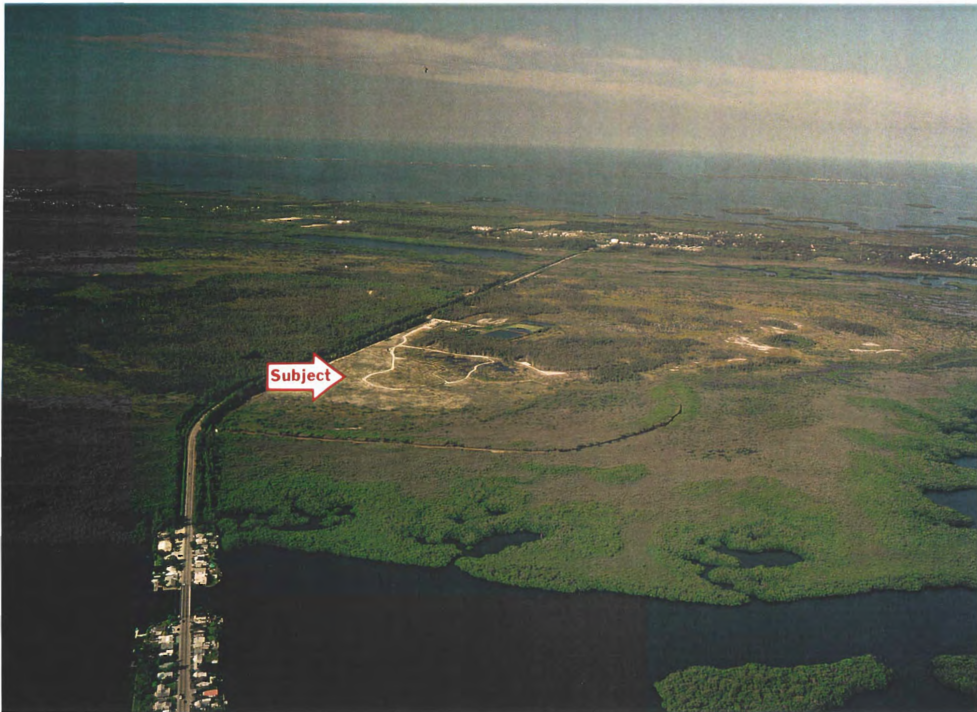
SEPTEMBER 1997 - PHASE I EXOTIC VEGETATION REMOVAL COMPLETE AT LITTLE PINE ISLAND - VIEW FROM MATLACHA PASS AQUATIC PRESERVE
