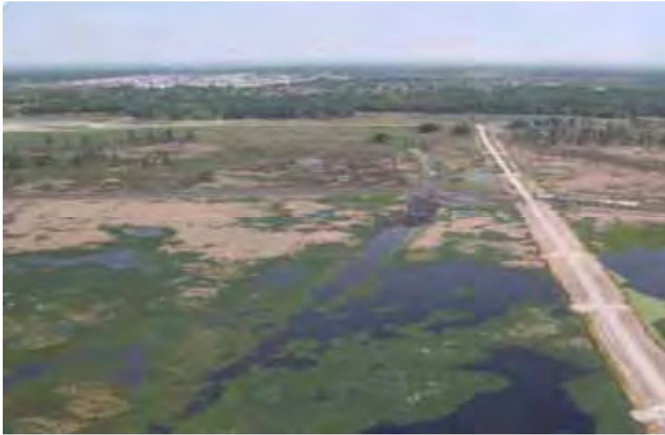
The 3,050 ft. long Center Road berm just after construction as sod is being installed on the slopes. To minimize the potential of sedimentation, the road berms were constructed prior to filling the western segment of the Banana Creek Canal and contributing ditches. An open water component west (left) of the Center Road is heavily used by water fowl, wading birds and alligators.
