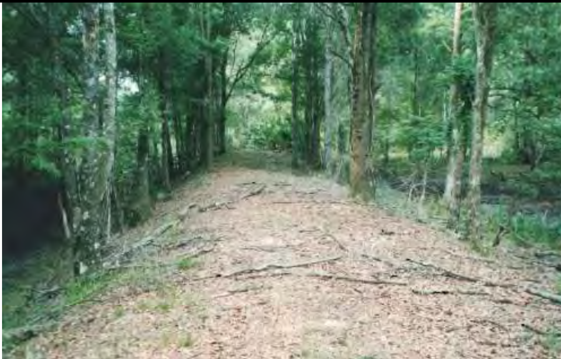
Pre-Construction - Site 4 (2005) – the northern half of the abandoned tram berm crossing the Pithlachascotte River wetland floodplain, blocking and diverting flow to the river channel instead of downstream wetland floodplain habitat.
