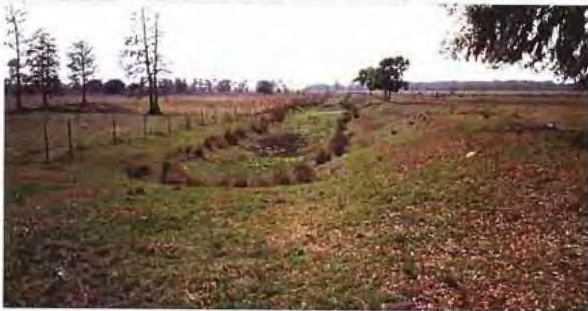
View south from the north end of the remnant and unstable Center Road and adjacent ditch that diverts and drains water south to the Banana Creek Canal. The ditch will be backfilled and clean fill used to reconstruct and elevate the road to restore west-east sheet flow hydrology and adjacent marsh habitat.
