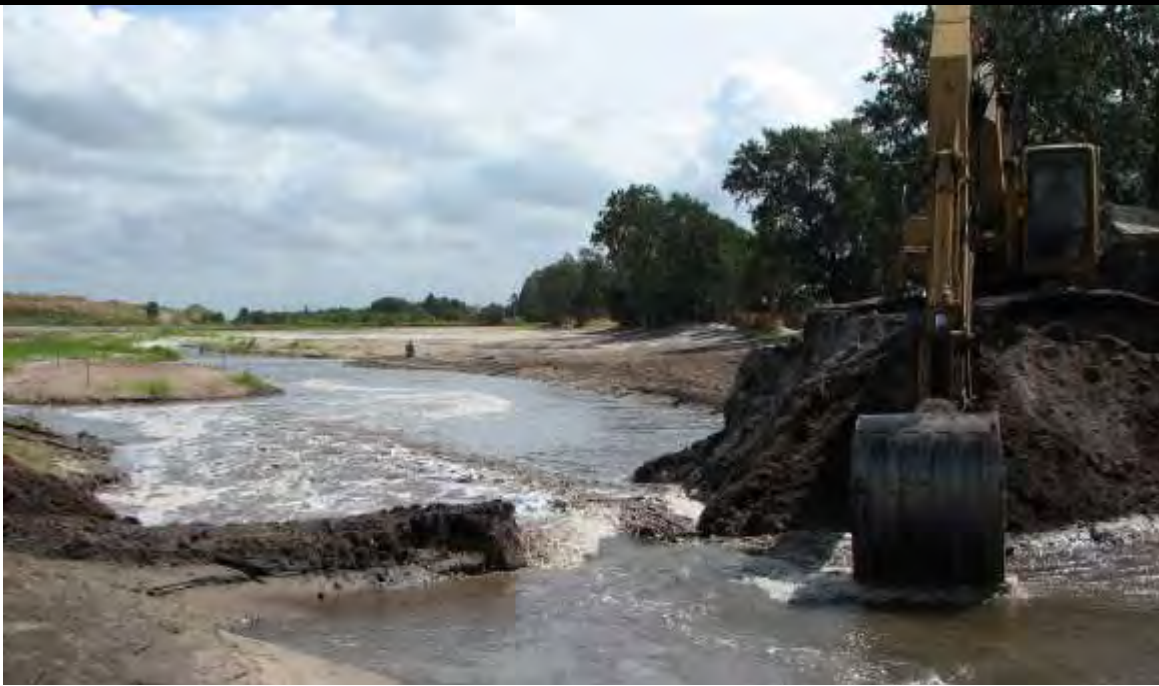
Marsh grades are final and the backhoe breaches the canal block to open tidal connection and flow into the constructed wetland.
