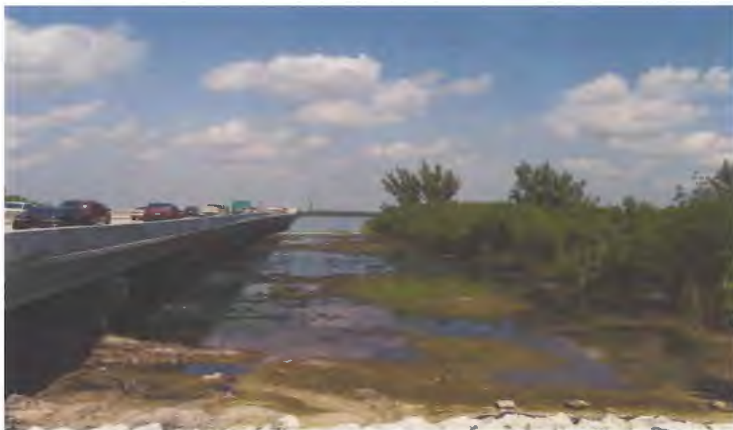
Site C – Post-Construction (Sept. 2003) – the new northbound bridge has been constructed and old bridge removed, exposing bare soil that was under the bridge. The area was planted with white mangrove, black rush and saltmarsh bulrush.
