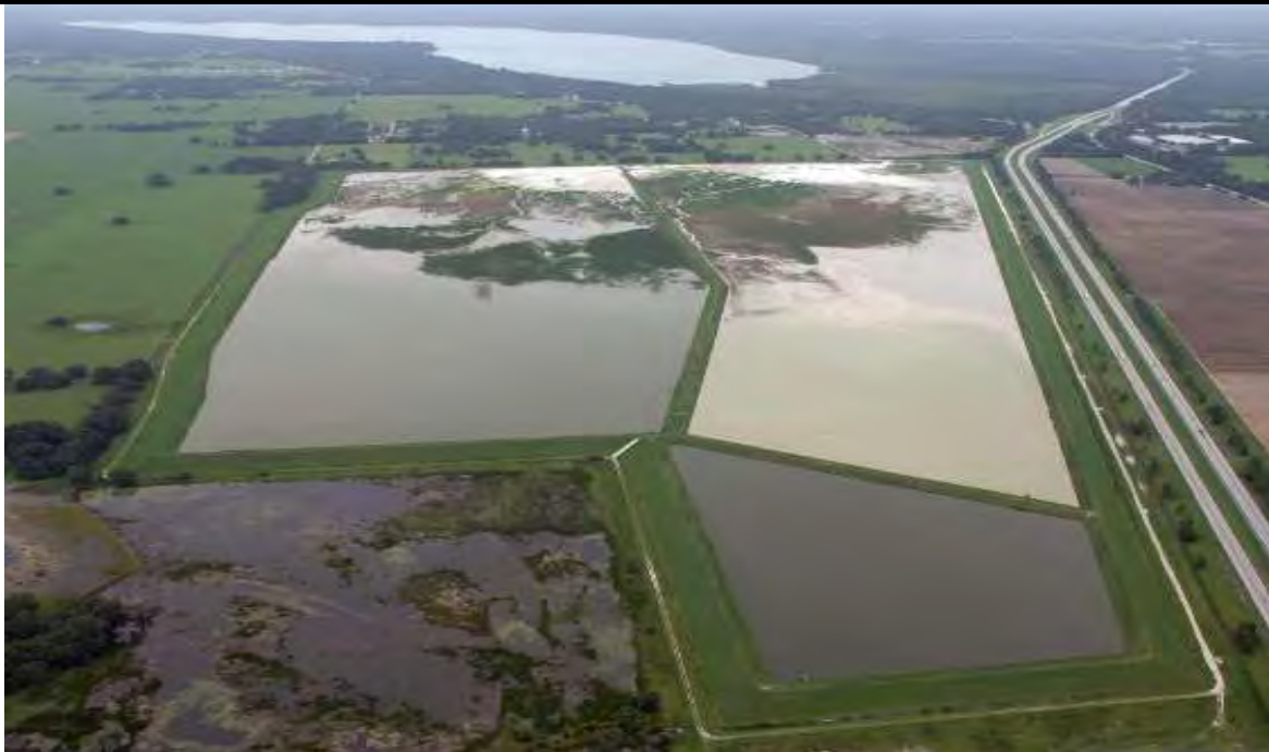
Aerial view of the sediment disposal cells constructed south of the lake (top of photo), the I-75 bridge wetland crossing being mitigated with this project is on the top right side of the photo.
