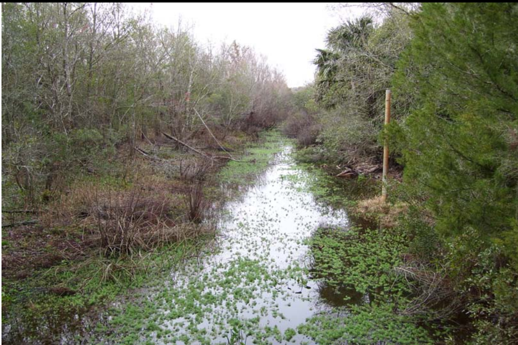
Shinn Ditch - View south from atop the wooden bridge crossing; the bridge will be removed and replaced with the construction of Ditch Block #4 wet crossing that will still allow vehicle access but detain water from discharging north into the Withlacoochee River. Berm spoil material along the bank will be used to fill the ditch and a low gradient sediment sump will be graded along the upstream side of the block.
