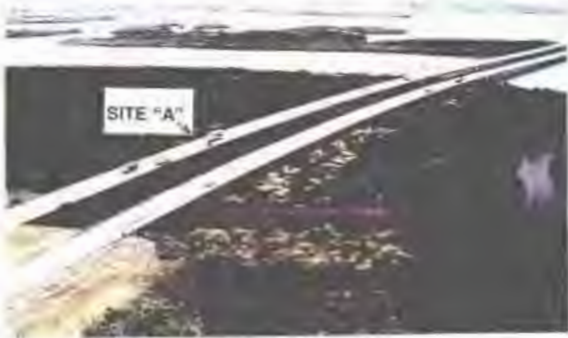
View of Interchange
