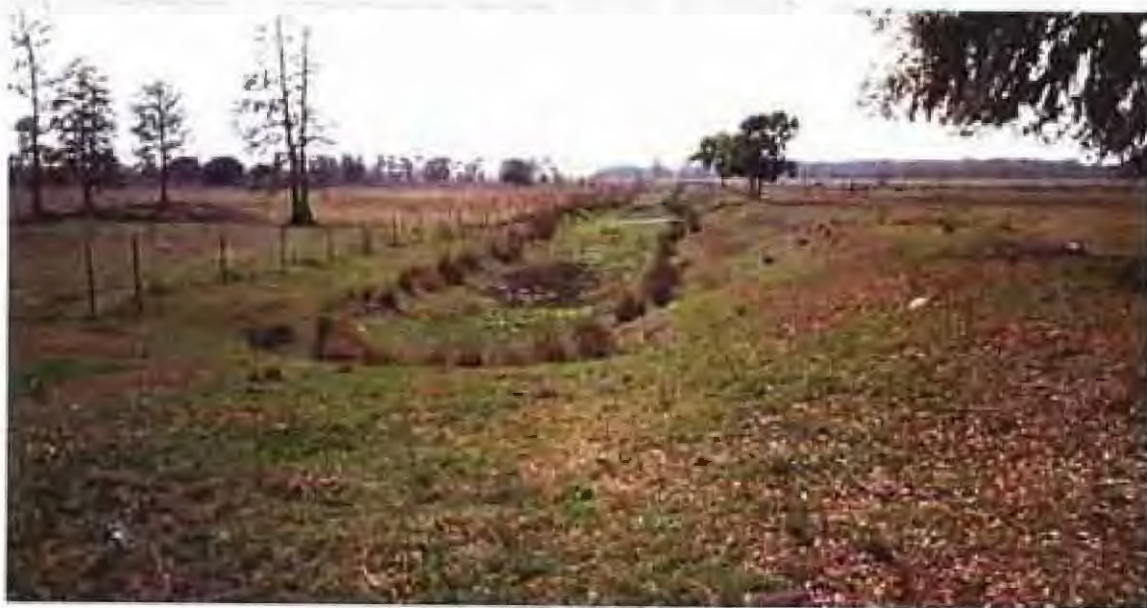
View south from the north end of the remnant and unstable Center Road and adjacent ditch that diverts and drains water south to the Banana Creek Canal. The ditch will be backfilled and clean fill used to reconstruct and elevate the road to restore west-east sheet flow hydrology and adjacent marsh habitat.
