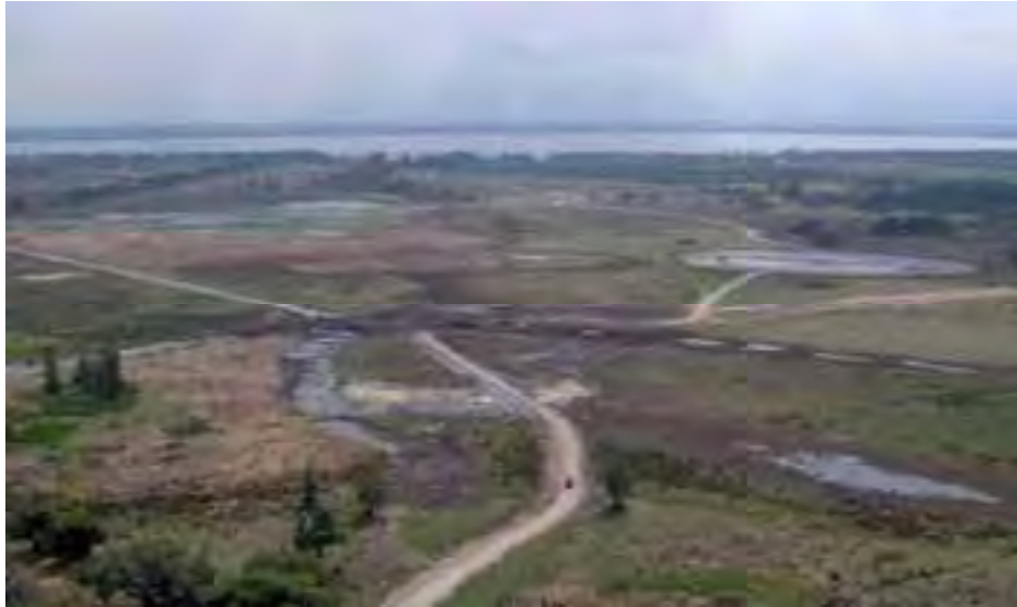
The West Road was historically a dry road crossing at natural grade over the pasture. The new road is within the same footprint and still at natural grade, but was reconstructed with crushed concrete. The majority of the road is now below the surface water elevations, maintaining a wet crossing used by vehicles only when necessary. Backfilling of the Banana Creek Canal and contributing ditches are evident (right to left), conducted just prior to removing the western levee to restore flow.
