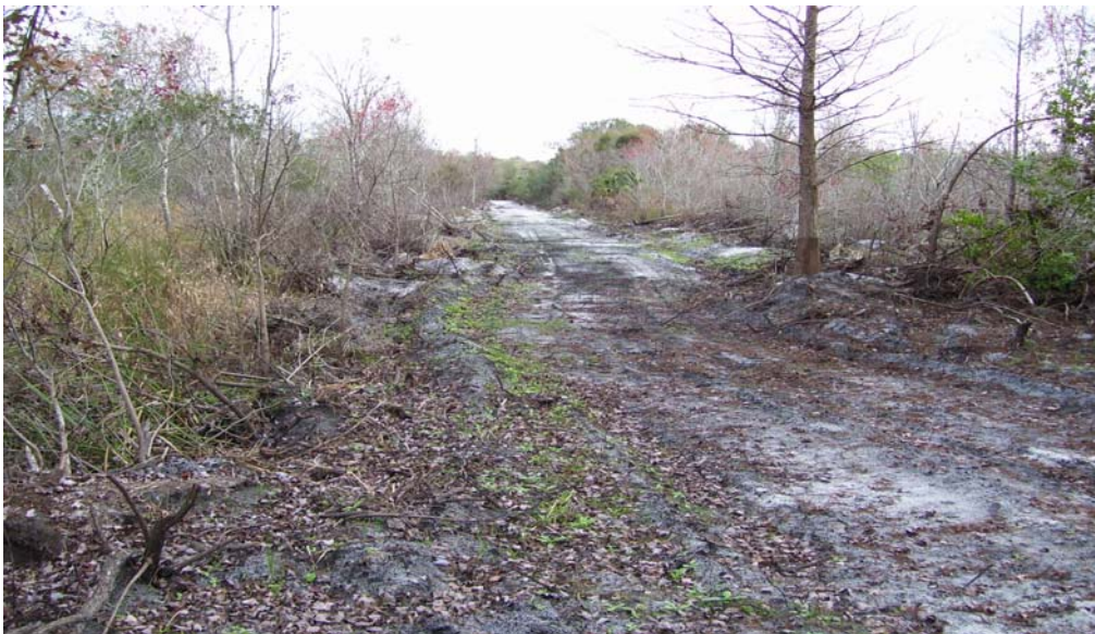
Shinn Ditch Access Road Berm - View north along the berm from area of proposed Ditch Block #2 (Shinn Ditch to the left). Constructing the four blocks and breaching the adjacent berm will aid in restoring sheet flow hydrology and appropriate hydroperiods for the drained wetland habitats.
