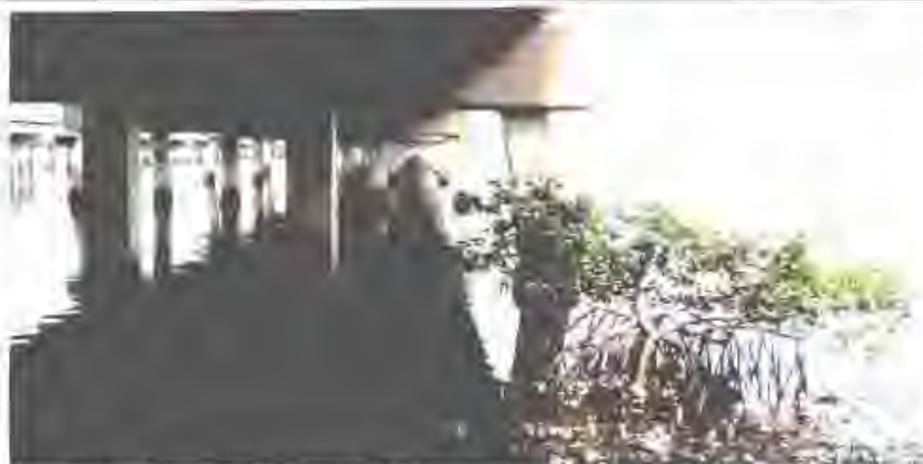
Site C - View from the southern shoreline of the Peace River, underneath the northbound bridge proposed for removal. Some red mangrove along the banks, seagrass beds within the river will not be impacted by bridge construction.
