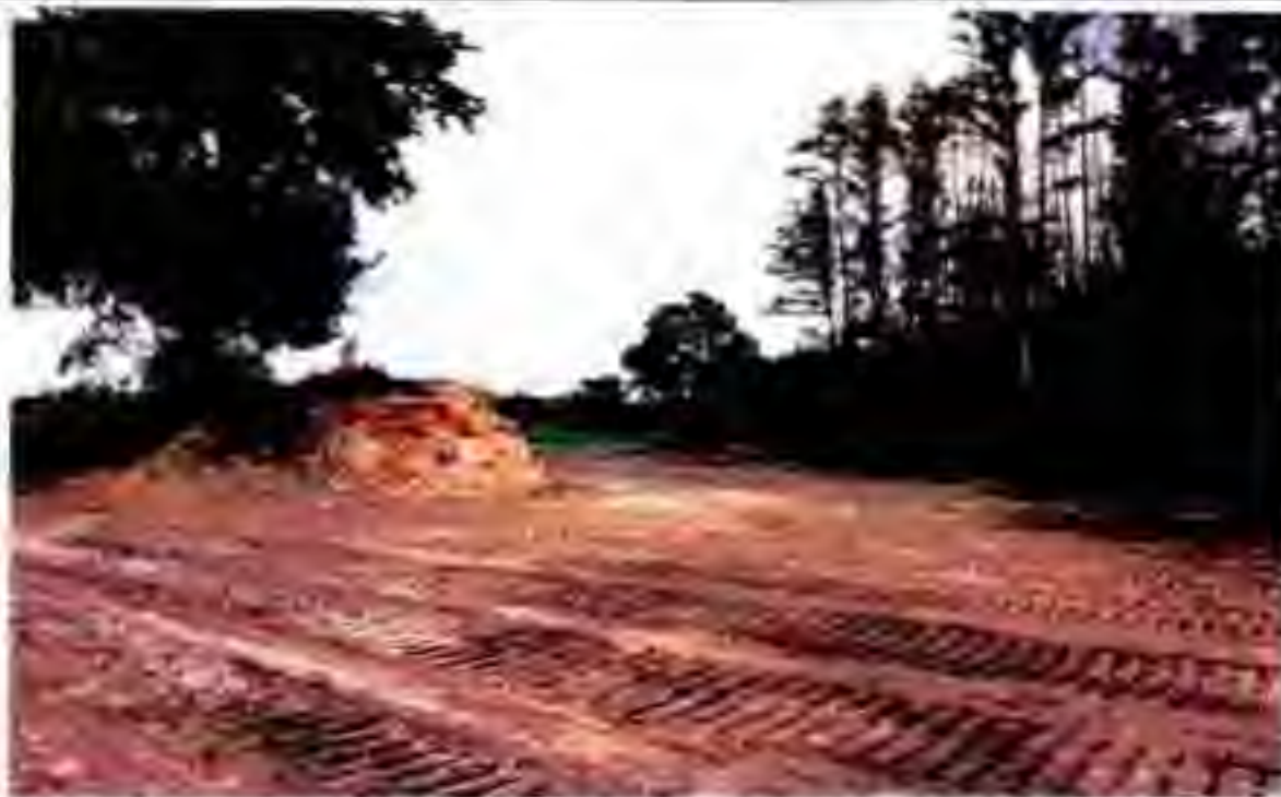
Same view as above photo after spoil material was backfilled. Preserved oak tree (left) on top of spoil mound depicts the amount of graded material required to fill the perimeter ditch.
