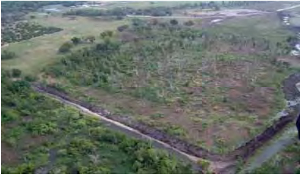
View from the western boundary of the property looking east. The north-south levee (900 ft. long, avg. 5 ft. tall) has just been backfilled into the adjacent ditch to restore western water sheet flow through the remnant forested wetland and proposed forested wetland restoration area. View of a backfilled portion of the Banana Creek Canal is evident along the right side of the photo.
