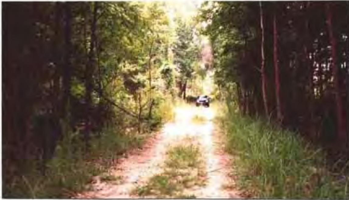
Site 2 – View of access road berm crossing through the Pithlachascotee River floodplain, the majority of this crossing's sideslopes are stabilized.
