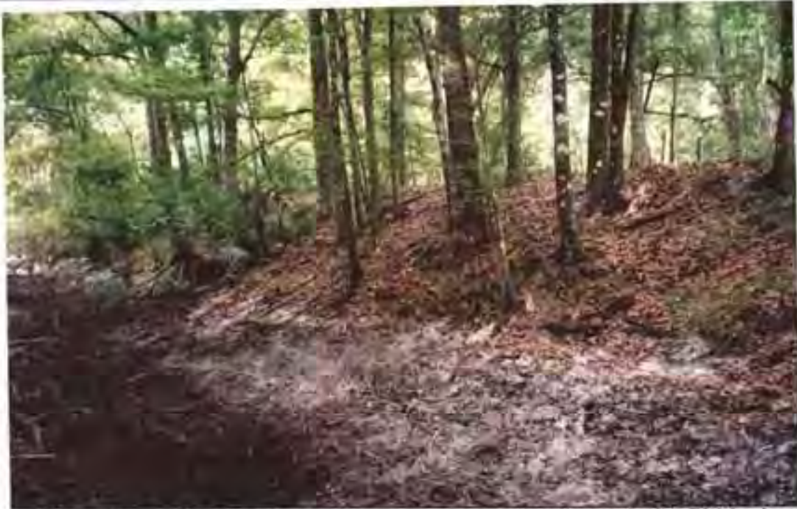
Site 4 – Side view of the abandoned tram berm crossing through the Pithlachascotee River floodplain. Breached berm material will be placed within dredged donor area (left), which will elevate and restore the historic floodplain grade.
