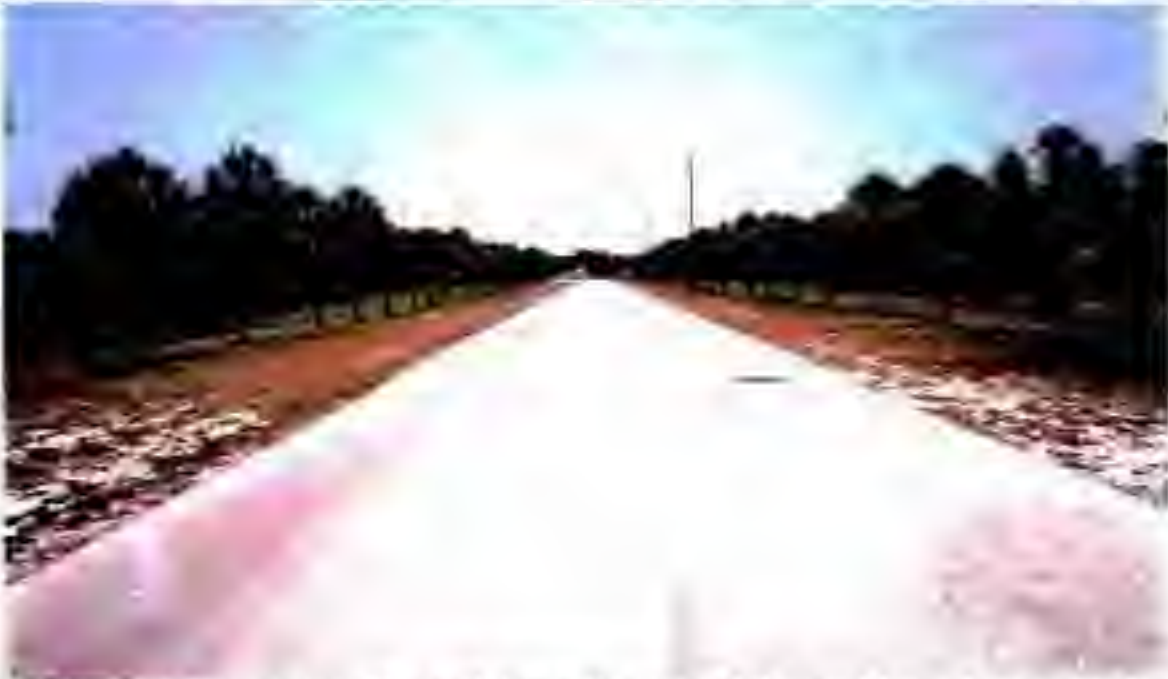
View of the maintenance road, north toward some of the park's maintenance facilities. This portion of the roadway will have to be slightly elevated to accommodate bridge height clearance.
