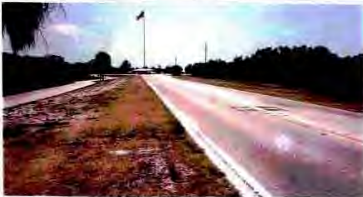
View of the entrance road (Pinellas Bayway) south toward the park's visitor center along Anderson Road. This portion of the roadway will have to be slightly elevated to accommodate bridge height clearance. Bicycle path to the left.
