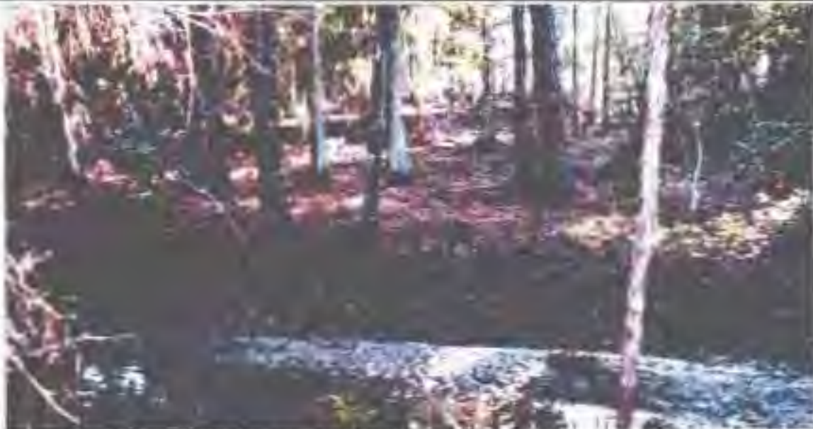
Bee Tree Drain – Adjacent to Monitor Site 22, the ditch drain (foreground) dewateres the adjacent forested wetland, allowing pines and laurel oaks to invade the system. The cypress lichen elevations indicate historic seasonal high water elevations but there are no indications that the water has overflowed the banks in many years. A ditch block along the downstream wetland boundary will restore the flow back through this wetland.
