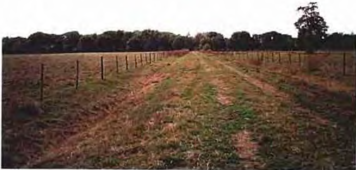
View south of the north portion of East Road where it crosses the northeast pasture. The Banana Creek Canal with trees on the adjacent spoil material is in the background. The road will be elevated and culverts installed to restore west-east surface water sheet flow and adjacent marsh habitat.
