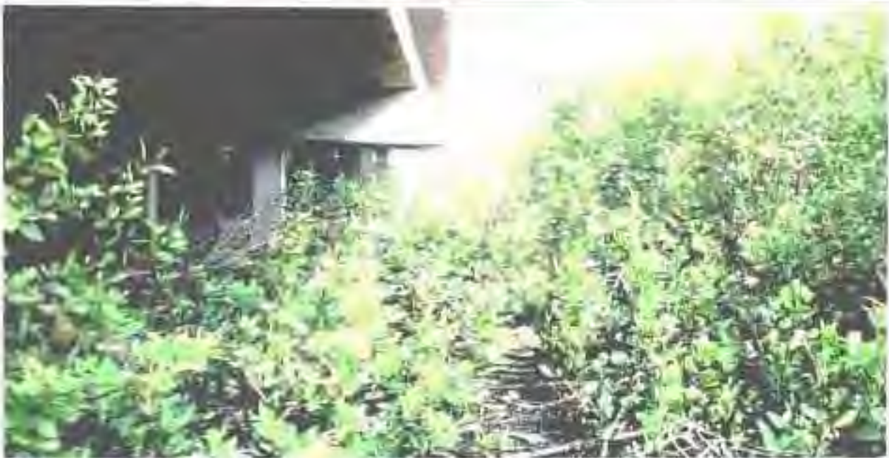
Site C - View of the temporary impact area (right) and proposed span removal (left). The temporary impact area is dominated by white mangrove, including shrub-size mangroves that have generated under the edge of the existing bridge span.
