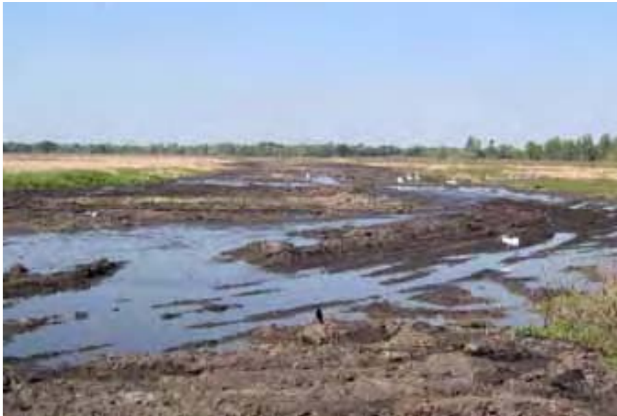
Same view of the Banana Creek Canal a week later, just after filling and prior to planting with herbs such as pickerelweed and arrowhead.
