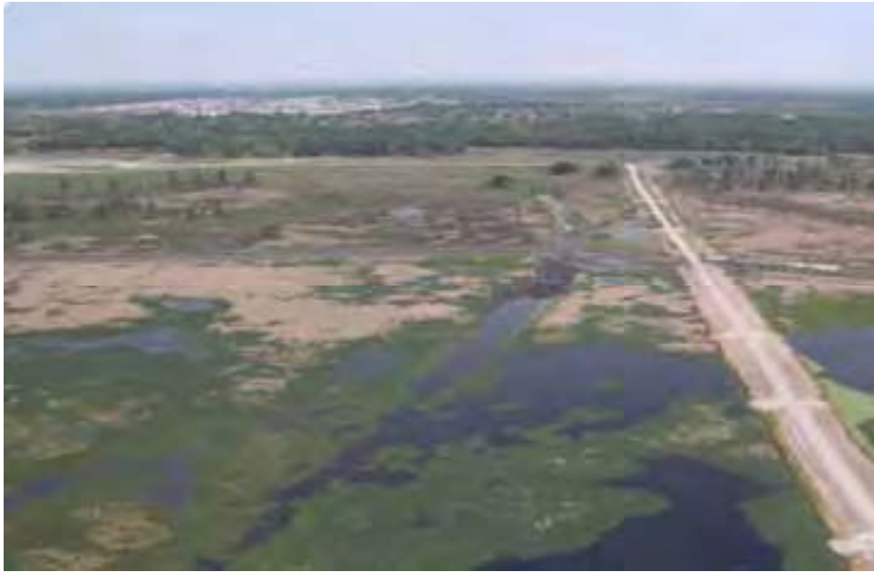
The 3,050 ft. long Center Road berm just after construction as sod is being installed on the slopes. To minimize the potential of sedimentation, the road berms were constructed prior to filling the western segment of the Banana Creek Canal and contributing ditches. An open water component west (left) of the Center Road is heavily used by water fowl, wading birds and alligators.
