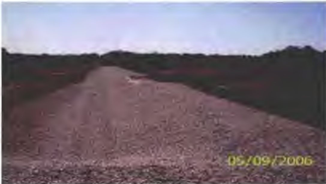
An 810-ft. long discharge weir was constructed to detain surface water, thus restoring the natural hydroperiod of a large slough wetland.
