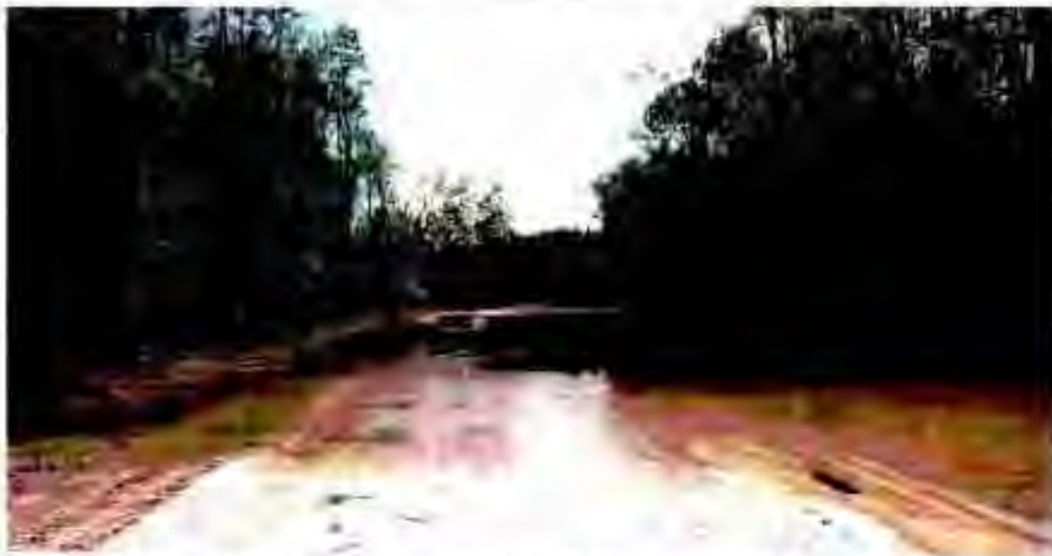
View of the filled east-west ditch and removed tram road, just after construction and prior to tree planting, wetland groundwater and surface water sheet flow hydrology is restored.
