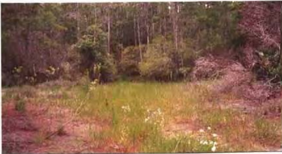
Site 8 – The ditch outfall area along the wetland/upland boundary is shallow and wide, a ditch block will be installed to remove the dewatering conditions caused by the ditch.
