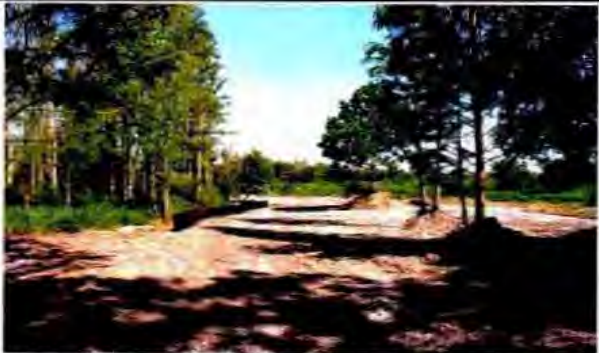
Same view as above photo after spoil material was backfilled. Silt screens installed to minimize erosion into the adjacent wetland while ground cover is establishing. Note where practical, construction worked around the drip line to preserve trees located on previous spoil ridge.
