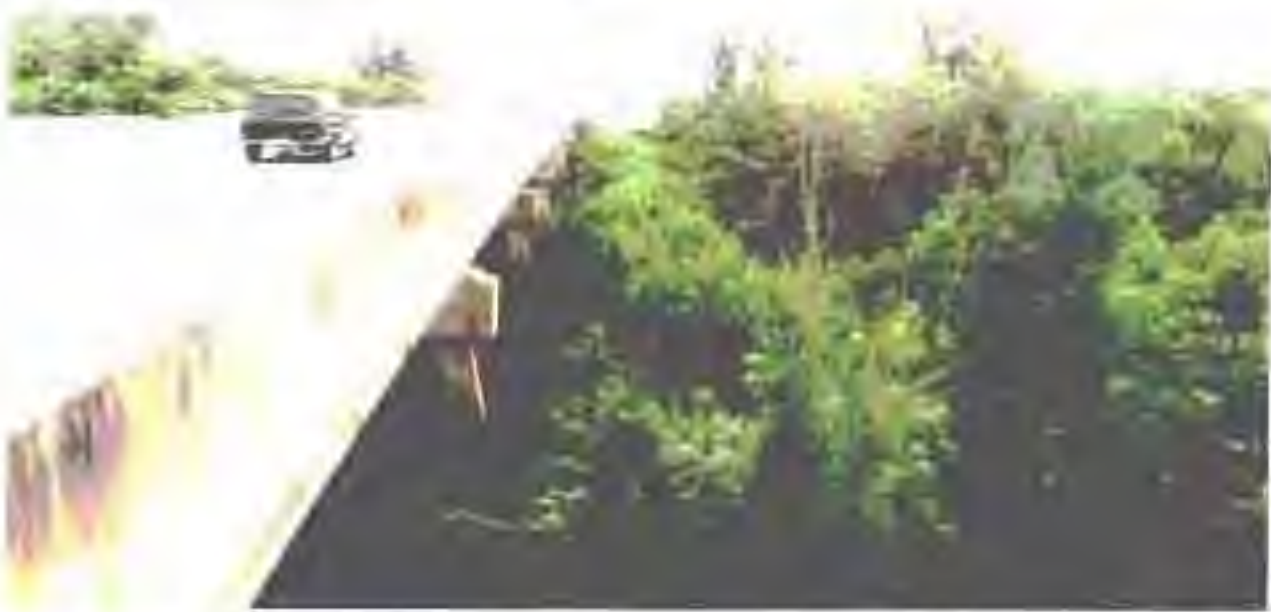
Site C - View from the northbound bridge's southern embankment, looking north at the proposed temporary wetland impact area associated with access of construction equipment. The temporary impact limits approximate the area where the mangroves are trimmed adjacent to the existing bridge span.
