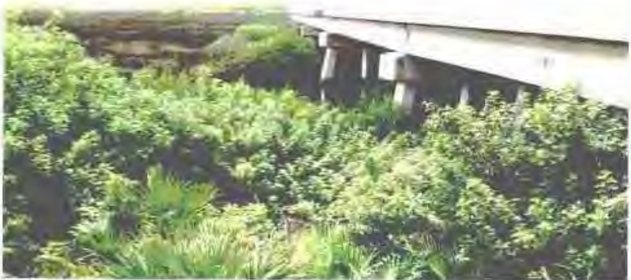
Site A - View from the northern bridge embankment area, looking south over the tidal branch (refer to Figure B for aerial depiction). Brazilian pepper along the embankment (foreground) with mangroves and black rush south of the open water and adjacent to the bridge.
