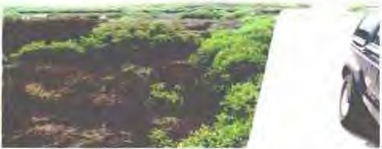
Site A - View from top of the northbound bridge, looking south at mangroves and black rush alongside the bridge within the proposed temporary impact area. These species will be planted to restore the temporary impact and to enhance a portion under the bridge span proposed for removal.
