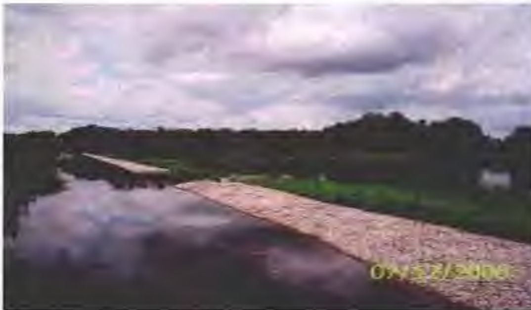
The discharge weir has a combination of two lower discharge elevations constructed with concrete, as seen above at the water overflow in the center of the weir. The broad "overflow" portion of the weir has limerock anchored within 6-inch geoweb containment system. A geotextile liner was placed under the rock to provide additional stability.
