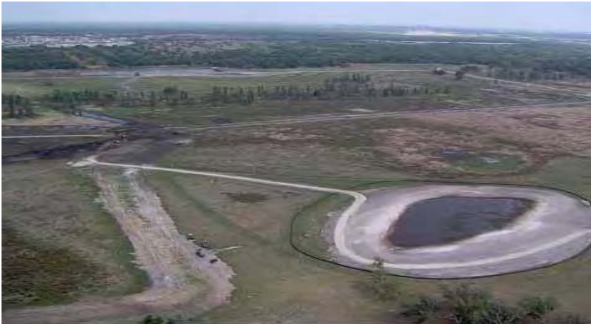
View of the finished Gator Pond, backfilled ditch (left), and Western Access Road during the late stages of construction. Construction equipment moving east to backfill the Banana Creek Canal (center).
