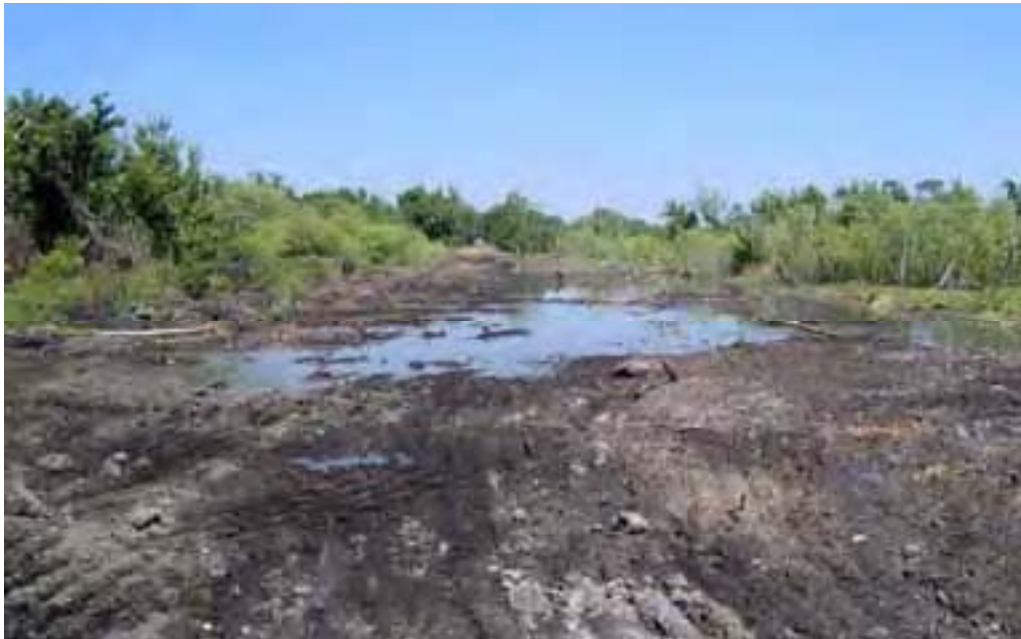
View from the southwest property boundary looking north at the footprint of where the levee was just pushed back into the ditch to restore sheet flow hydrology. The graded area was then planted with hydrophytic plants and trees.
