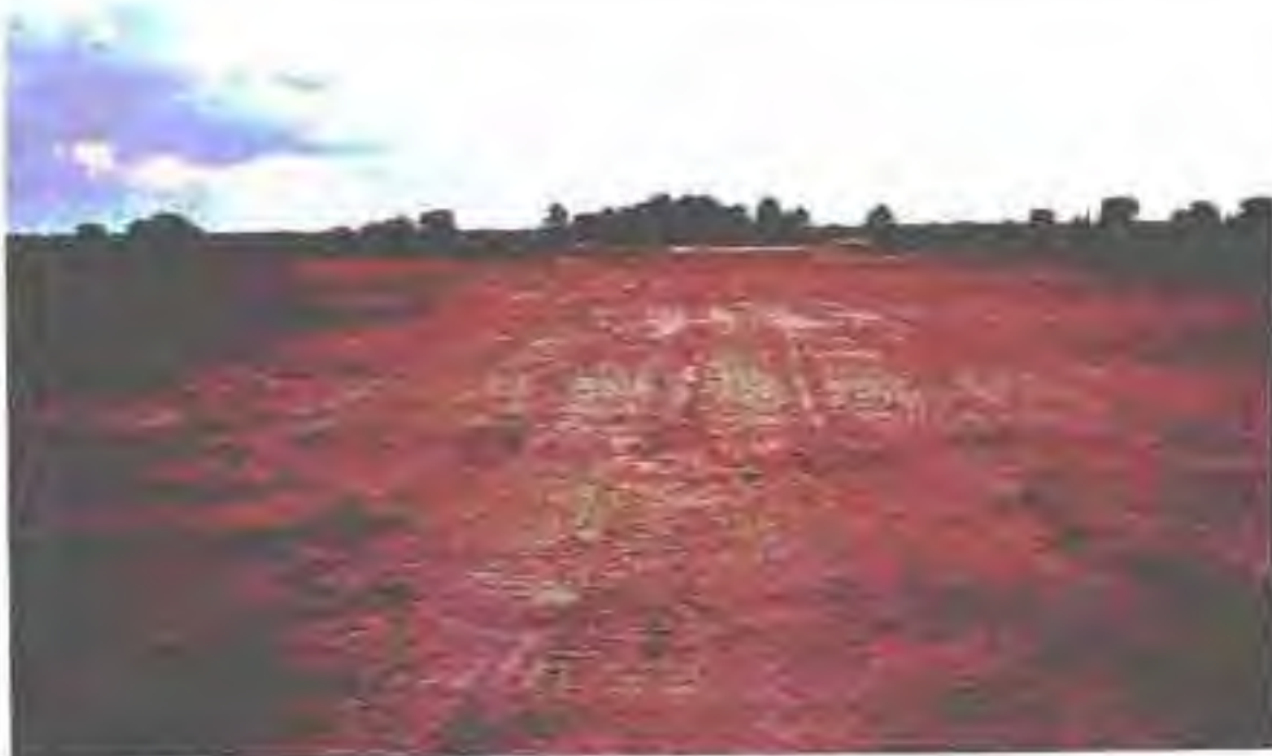
June, 2002 – Wetlands 5 & 6 – View from the east side of the marshes, looking west at the filled ditch (center) and graded spoil material (right) to restore hydrology.
