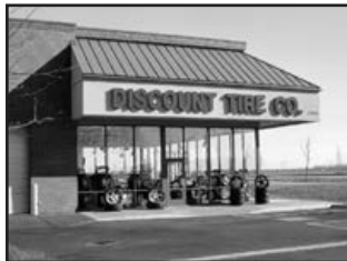
Low and mid-rise lifts can generally be found in tire shops, body shops and quick lubes.
