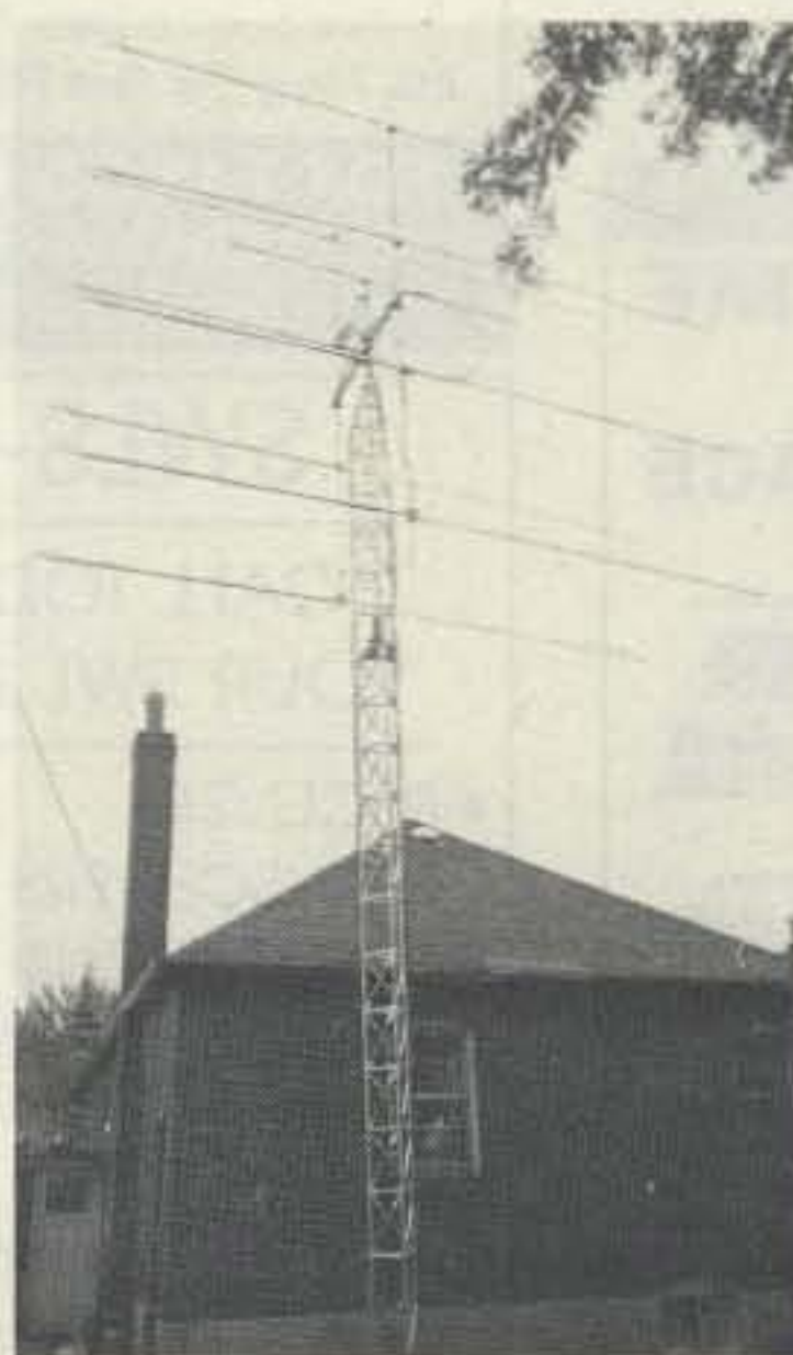
The EME array at VE3CRU. On 432, Hans uses 1.5 kW into eight 32-element yagis and has worked Australia, Japan, and Germany.
