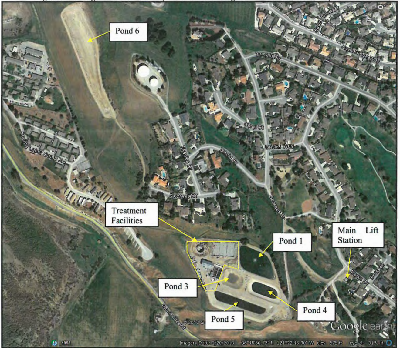
Figure 2-1: Ridgemark I Facilities (Photo taken during construction March 2013)
