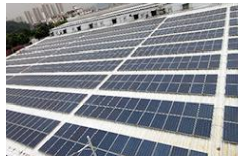
Solar panels installed on the roof (TRG in China)
