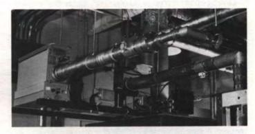
This TT50FL dual transmitter installation at WKYC-TV is the first in the country. Shown above are three TERMALINE "Reject Loads" with their THRULINE Wattmeters. The 50kW Test Load/Wattmeter is switched remotely (including water flow) from the studio 10 miles distant, where the reject power levels and main feed power are monitored (below left and right).
