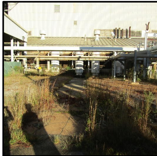
Waste Oil Facility
