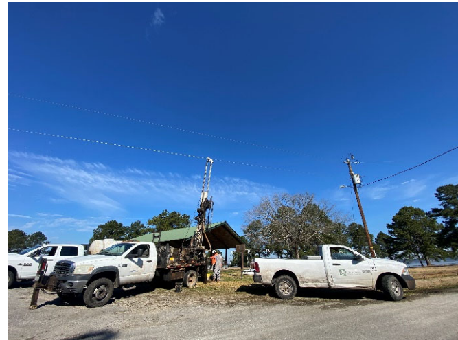
Facing Northwest at Boring B-03
