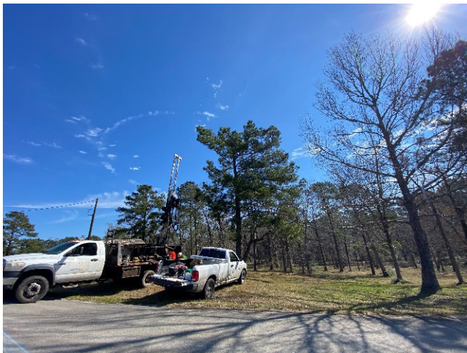
Facing East at Boring B-08
