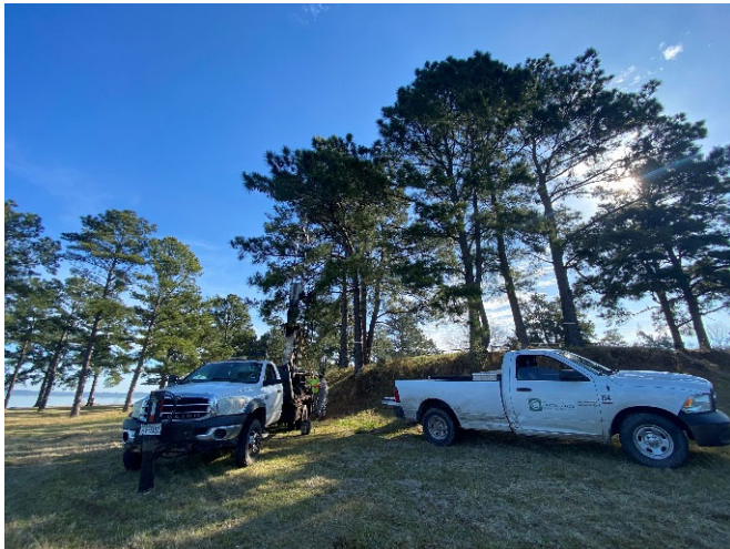
Facing East at Boring B-03
