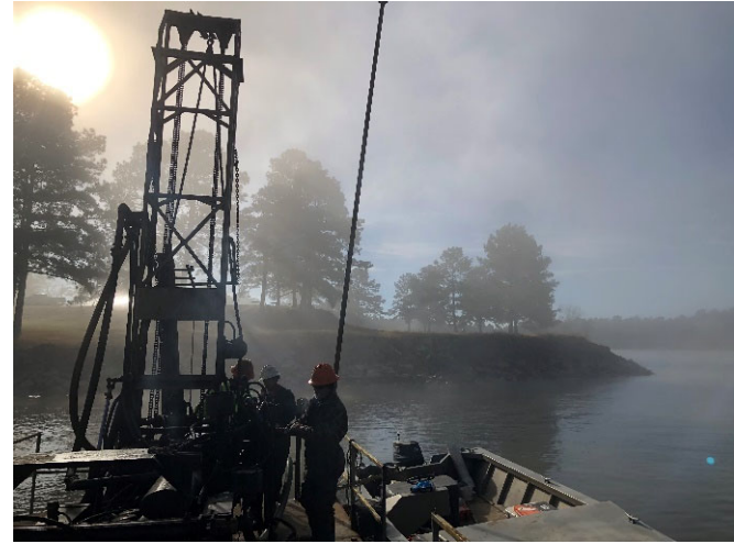
Facing Southeast at Boring B-16
