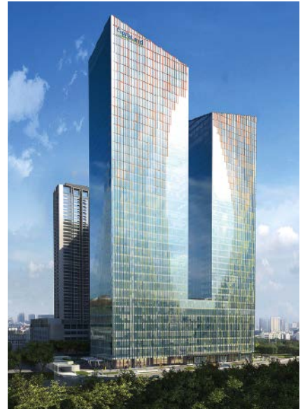
METROPOLIS OFFICE BUILDING HO CHI MINH CITY, VIETNAM
