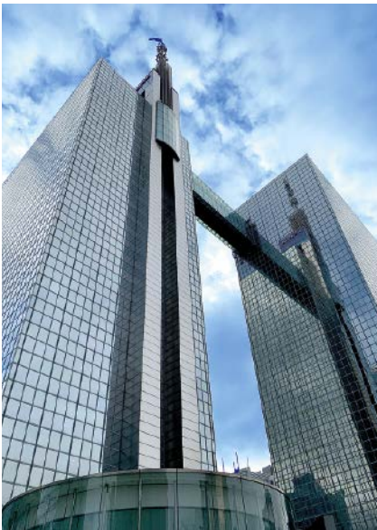
PROXIMUS CENTER BRUSSELS, BELGIUM
