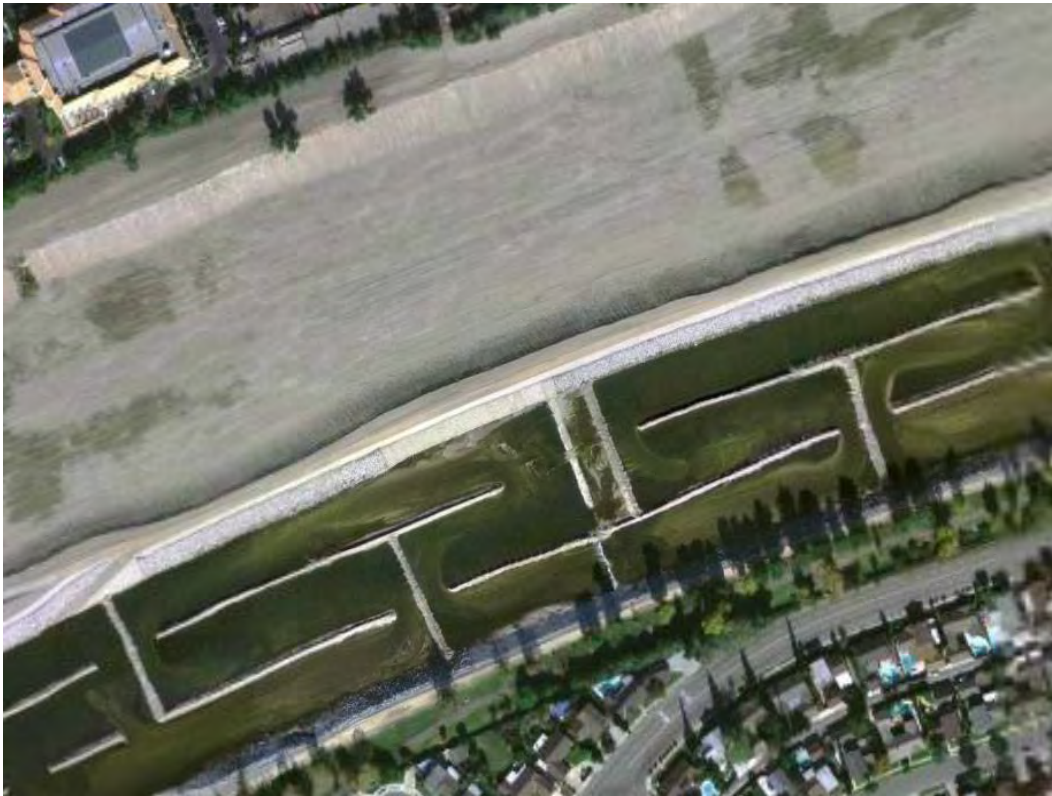
Figure B-2 Example of T&L Levees
