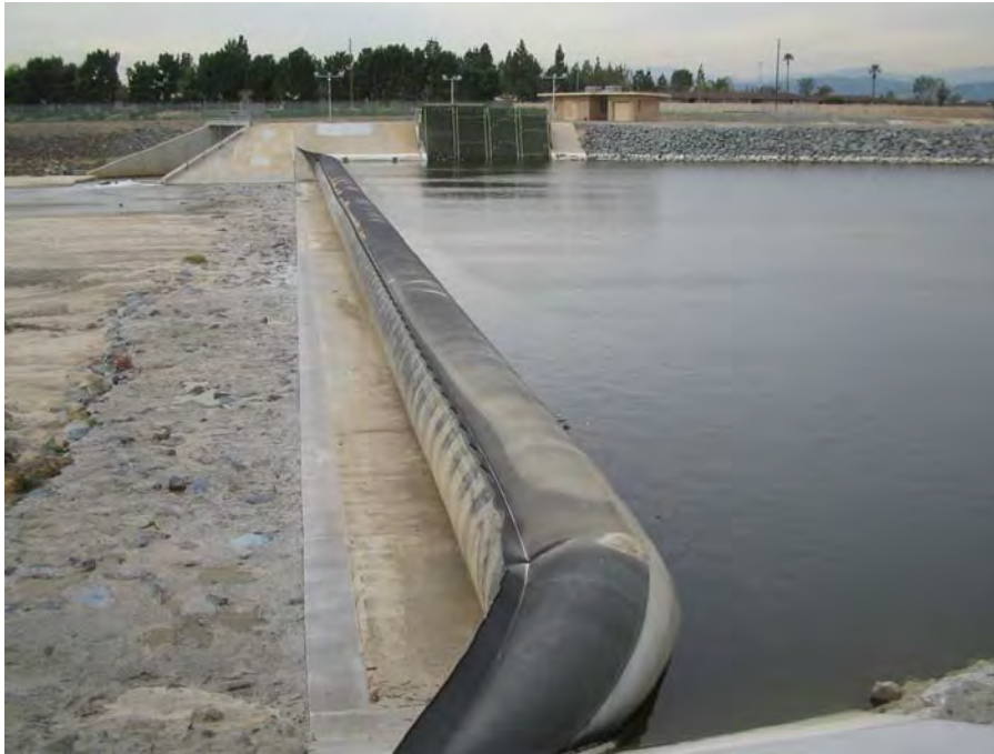
Figure A-4: Rubber Dam Structure Downstream of Glassell St.
