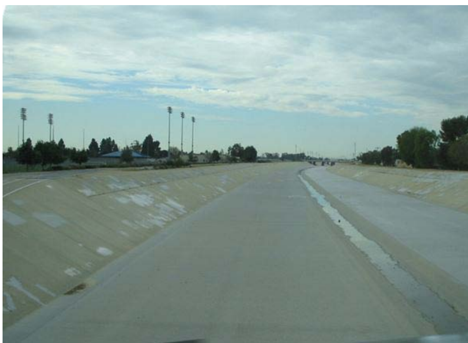
Figure A-10: Lined Channel Section at W. Edinger Ave. Looking Downstream
