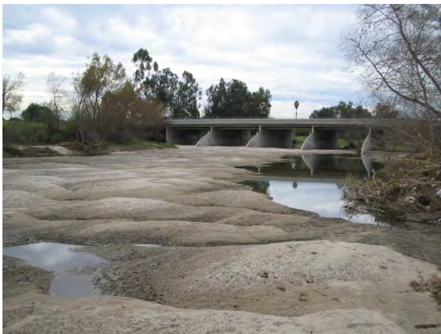
Figure A-8: Bed Material Upstream of Memory Ln. Bridge Looking Downstream
