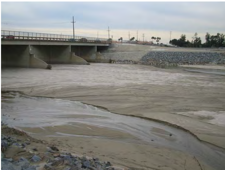
Figure A-7: Upstream of Chapman Ave. Bridge Looking Downstream Showing Mostly Sand Bed Material
