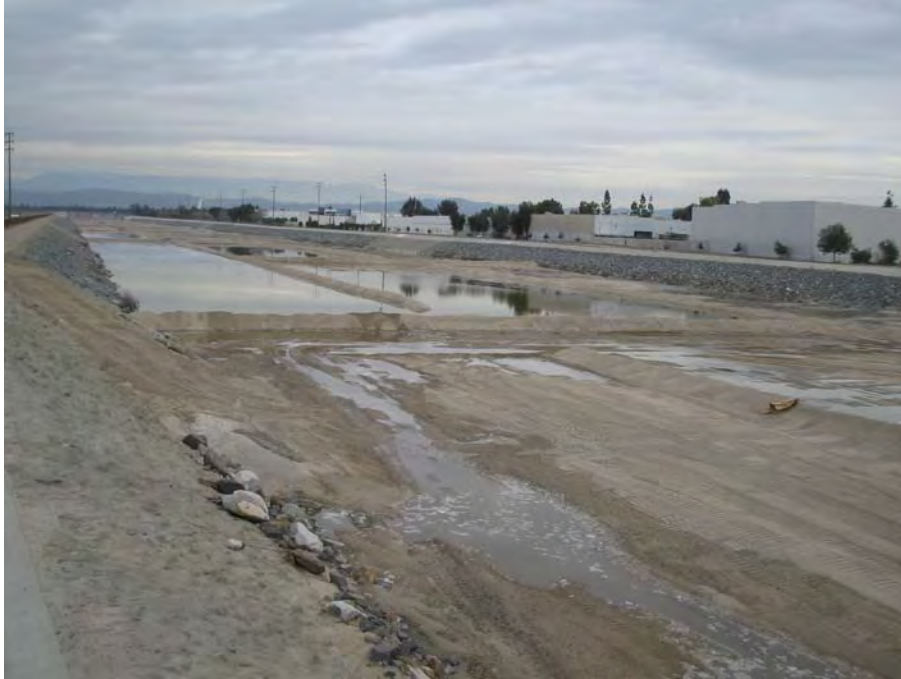
Figure A-6: Recharge Area Downstream of Orangewood Ave. Looking Downstream Showing Remaining Flow in River Detained by T&L Levees
