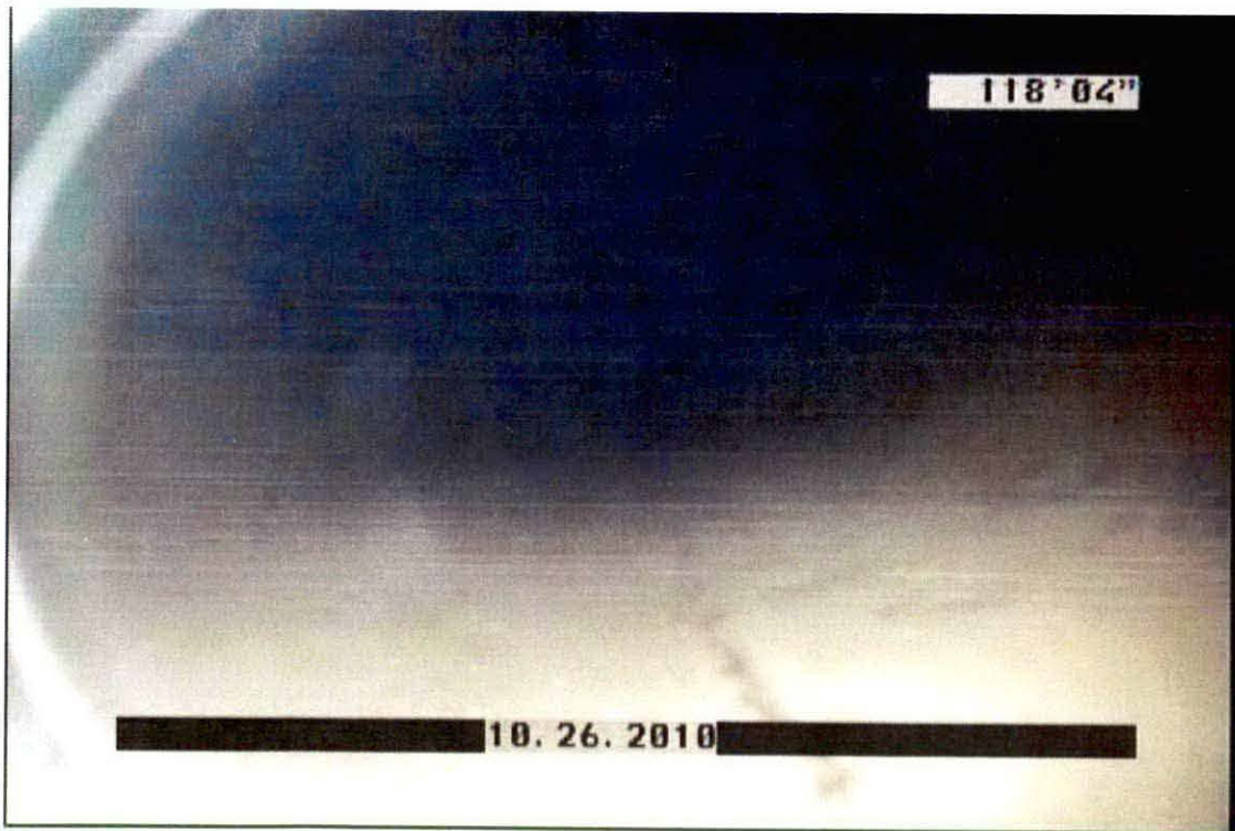
Figure 2. Image Captured by Video Inspection Rover
