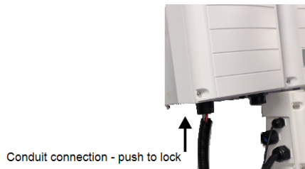
Figure 19: Connecting the conduit to the Secondary Unit
