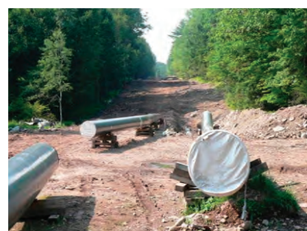
Pipeline construction in Pennsylvania.
