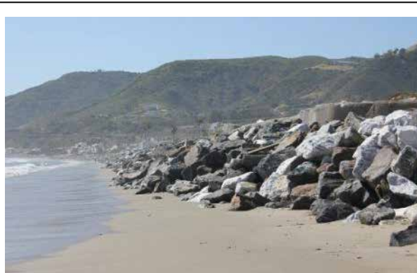
Illustration 3.6-3. The existing revetment rises up 12 to 15 feet in height above the low tide intertidal lands along Broad Beach, limiting public views landward from these public trust lands.
