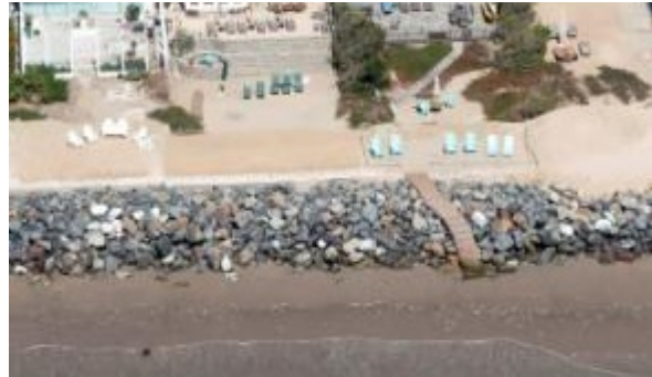
Illustration 3.2-4. Construction of the emergency revetment interrupted or blocked historic private vertical access to Broad Beach. In response, homeowners constructed, and appear to share, approximately 15 informal rock and geotextile bag stairways across the revetment. Waves have since damaged or eroded away some stairways.
