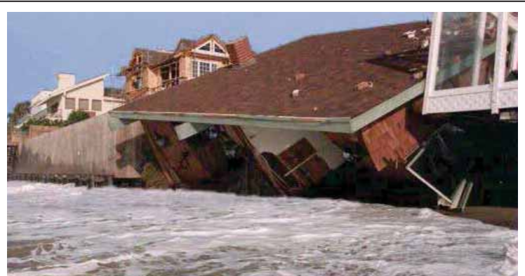
Illustration 2-2. Wave action in the 1997-1998 El Niño led to major structural damage to one Broad Beach home (source: Norton Karno, February 1998).
