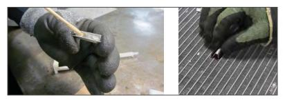
17. Lightly "crimp" the aluminum wrapper with needle nose pliers.
