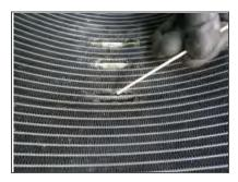
14. The vacuum pump should be able to pull the epoxy through the cut area to form a shape that works as a plug.
