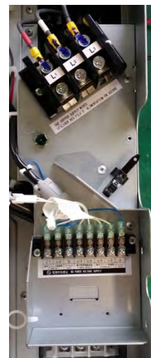
Close-up view of terminal block sub-assembly
