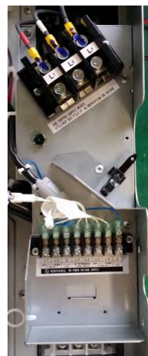
Close-up view of terminal block sub-assembly
