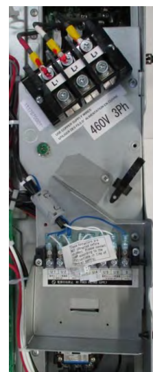
Close-up view of terminal block sub-assembly
