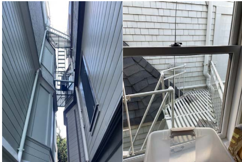
Photos of Fire Escape 1
