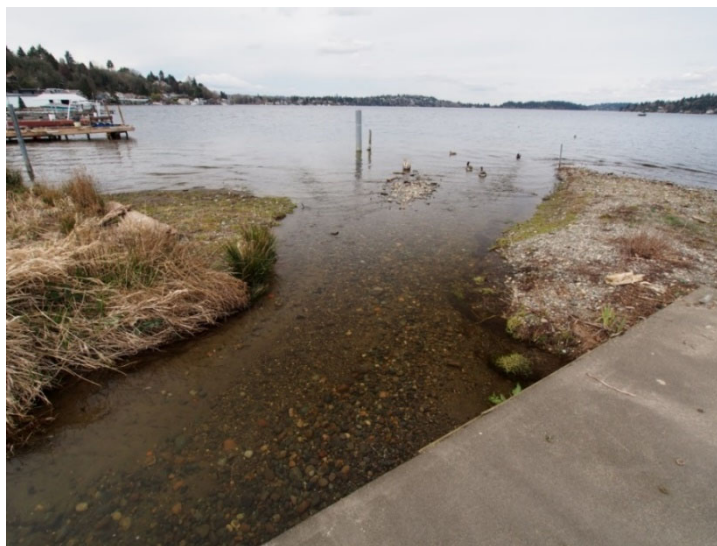
FIGURE 4.- Photo of the mouth of Taylor Creek and delta habitat with Lake Washington in the background. The concrete slab in the bottom right of the photo is severely undercut and was consistently used by juvenile Chinook salmon. Photo taken 3/23/2017 by Roger Tabor.
