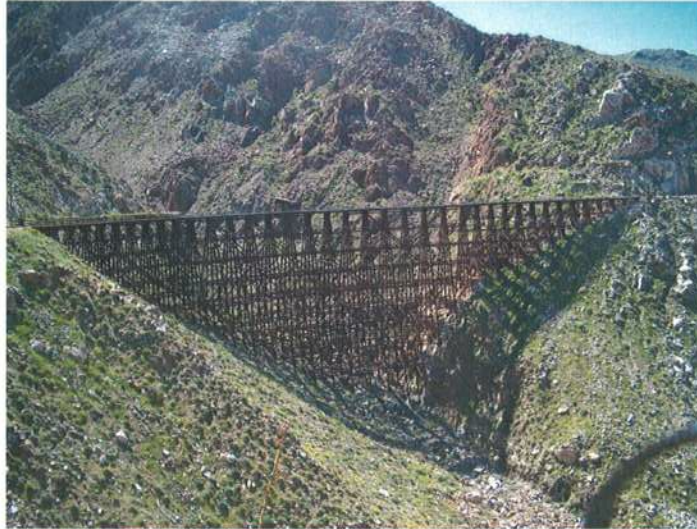
Goat Canyon Trestle Looking South
