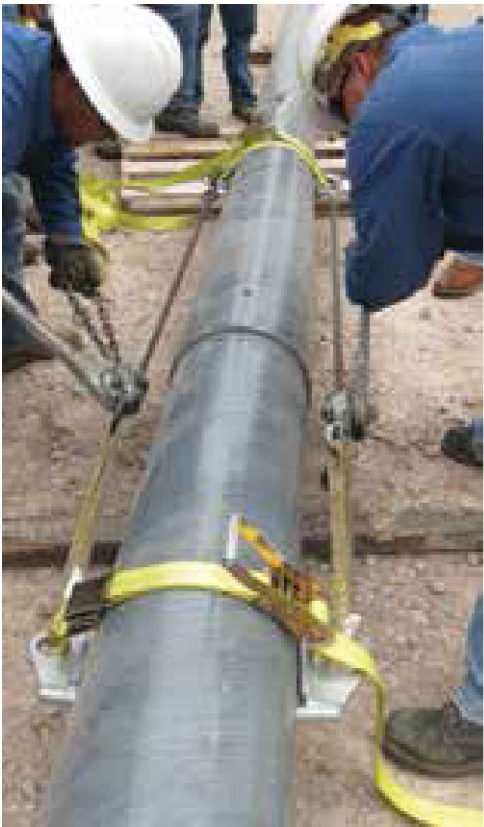
FIGURE 12 COME-ALONG INSTALLATION
