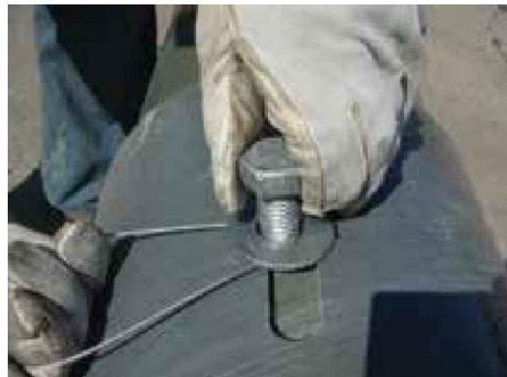
FIGURE 15 BOLT AND WASHER INSTALLATION
