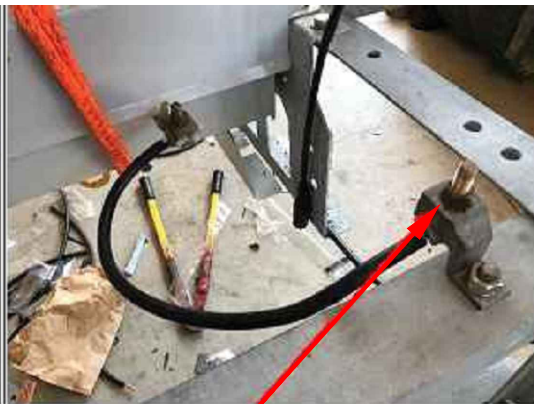
GROUND SWITCH FOR SWITCH FRAME
