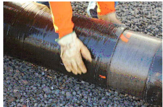
FIGURE 8 ALIGNING SECTIONS (J)
