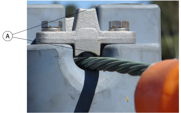
FIGURE 2 INCORRECT INSTALLATION
