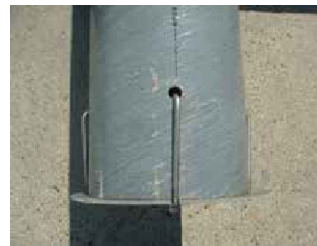
J-BOLTS ON OUTSIDE OF MODULE
