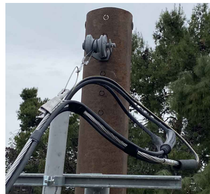
FIGURE 4 STORM SAFE FLEXIBLE BAIL ASSEMBLY
