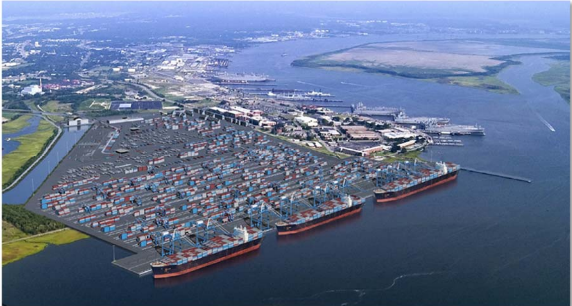
Figure 2-11: Rendering of the Hugh K. Leatherman, Sr. Terminal at Port of Charleston
