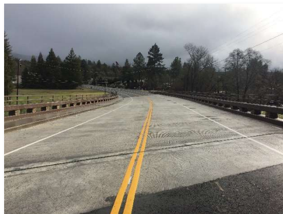
Figure 2.7 – Bridge Deck in Good Condition Morgan Territory Road, Contra Costa County
