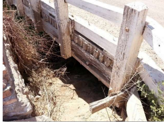
Figure 2.4 - Poor Superstructure and Substructure Condition Rating example Verde School Road over East Highline Canal in Imperial County, CA
