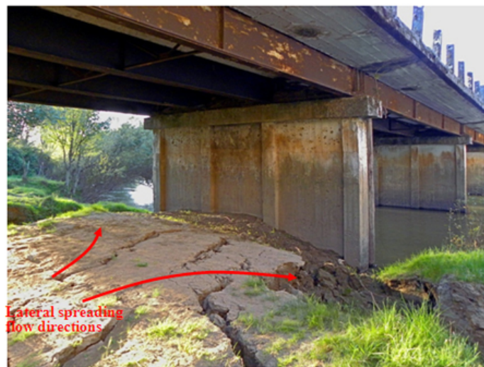
Figure A.11 - Soil liquefaction and soil lateral spreading
