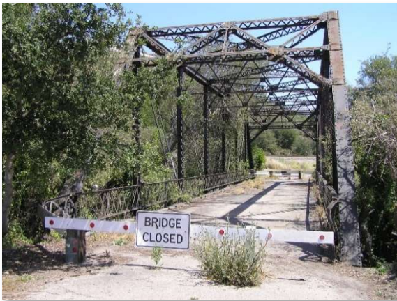
Figure 2.5 - Poor Deck and Superstructure Condition Rating example Bello Street Bridge over Pismo Creek in the City of Pismo Beach
