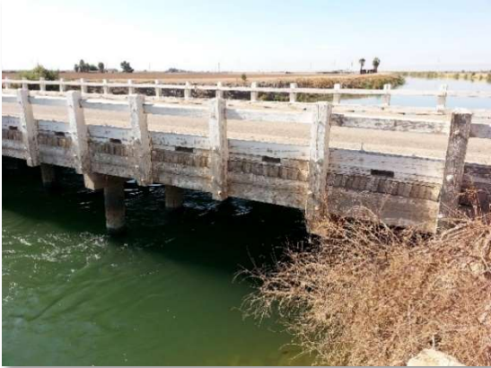
Figure 2.4 - Poor Superstructure and Substructure Condition Rating example Verde School Road over East Highline Canal in Imperial County, CA
