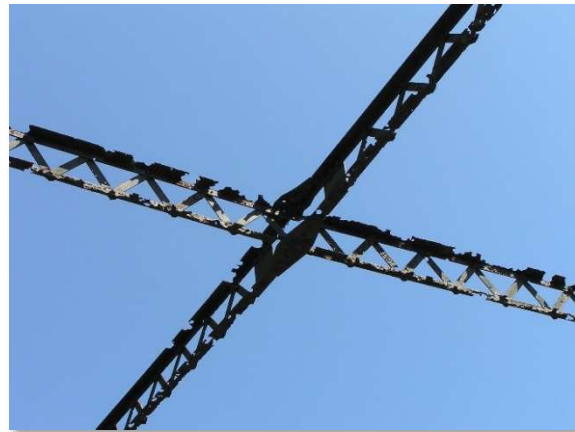
Figure 2.5 - Poor Deck and Superstructure Condition Rating example Bello Street Bridge over Pismo Creek in the City of Pismo Beach
