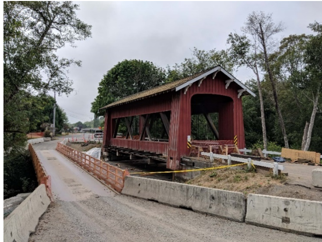
Figure A.8 - Potentially Historically Significant Timber Truss Bridge (Rehabilitated) Brookwood Drive over Jacoby Creek, Humboldt County, CA
