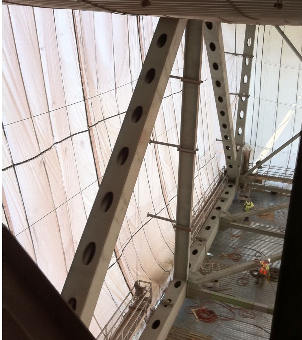
Figure A.10 - Containment System for Lead Abatement
