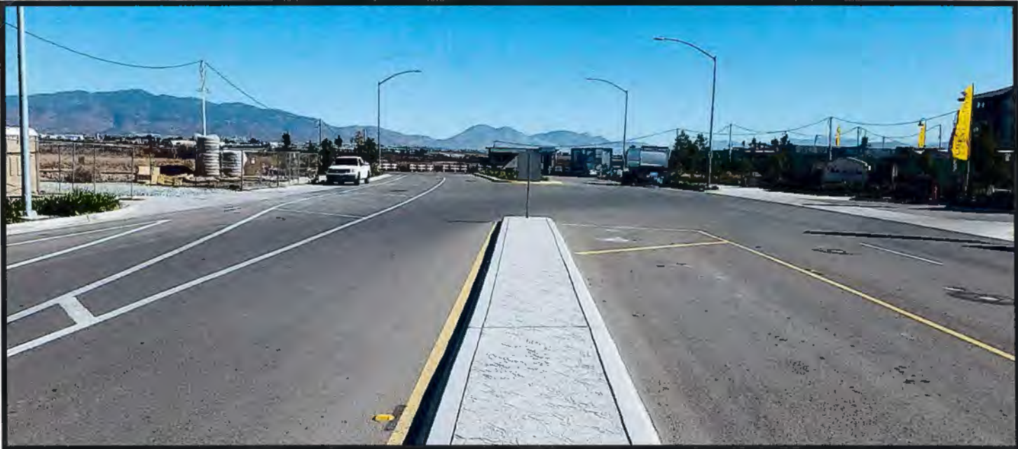
Looking east on Airway Road, toward cul de sac terminus located on western portion of site:
