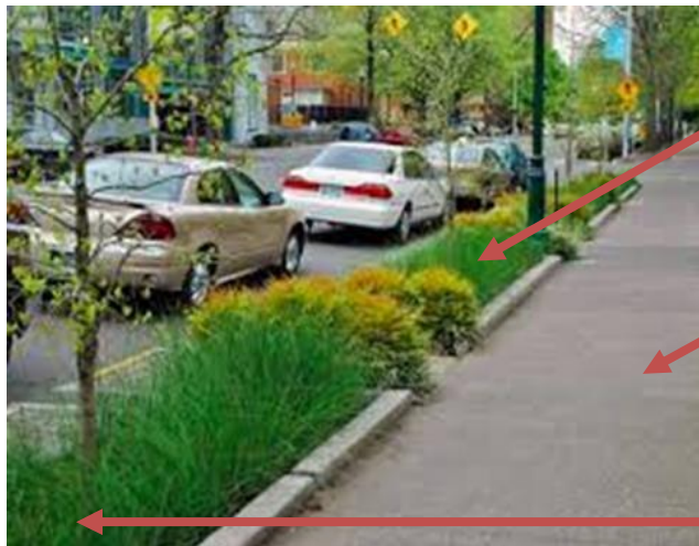
Figure 1: Illustration of Sample Structural BMP: Green Streets
