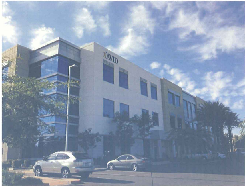
Looking at east elevation
