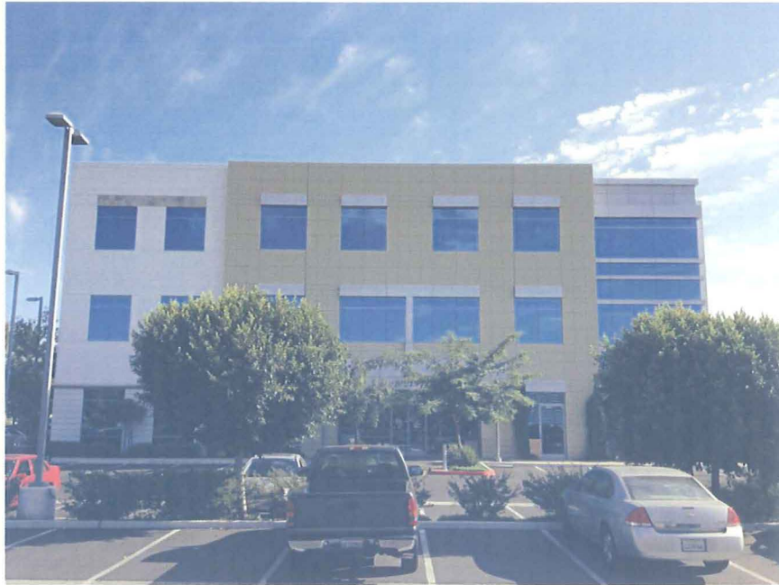
Looking at north elevation
