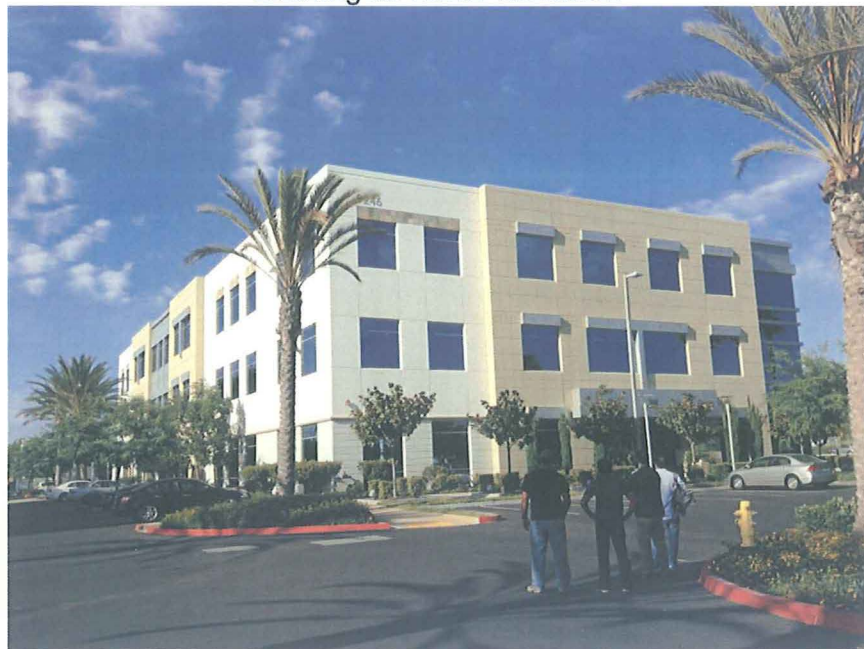
Looking at south & west elevation
