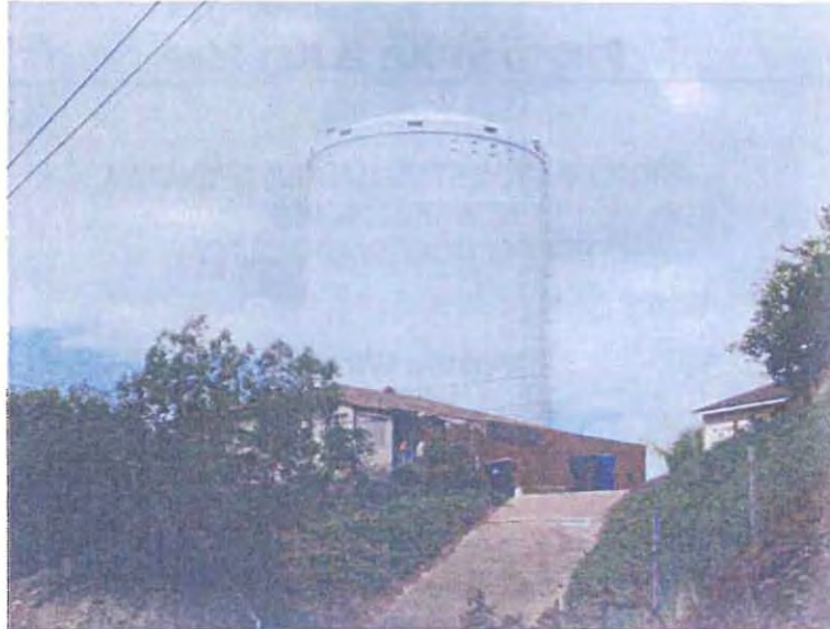
Looking northwest toward site
