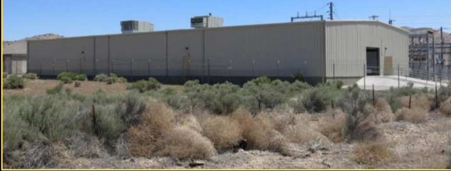
BESS facility at Monolith Substation
