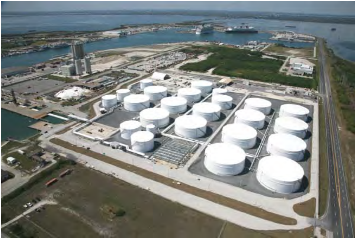
Figure 2-7 Seaport Canaveral Fuel Terminal
