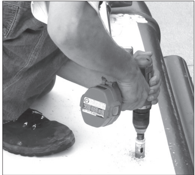
Figure 11 Drilling the Cable Access Hole
