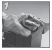
Insert CADWELD PLUS package into mold (optional: use with or without cover/baffle)
