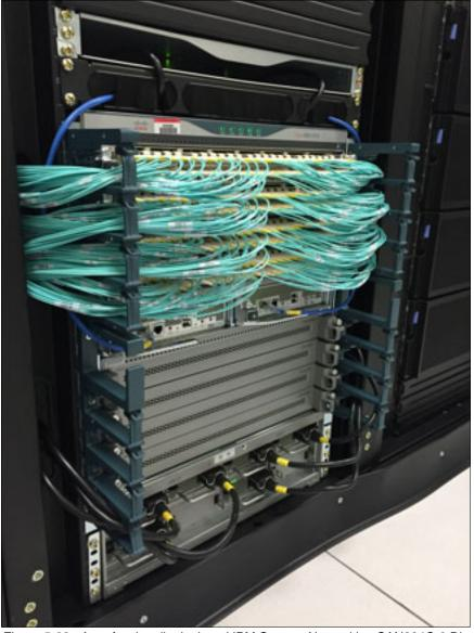
Figure 5-62 A professionally deployed IBM Storage Networking SAN384C-6 Director with plastic brackets in the front
