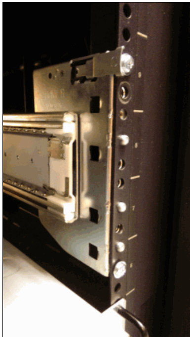
Figure 6-12 Installed outer rail member
