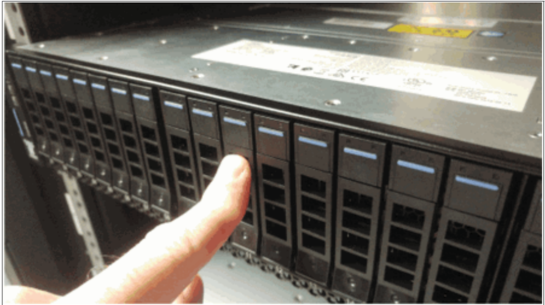
Figure 5-12 Completing the drive installation
