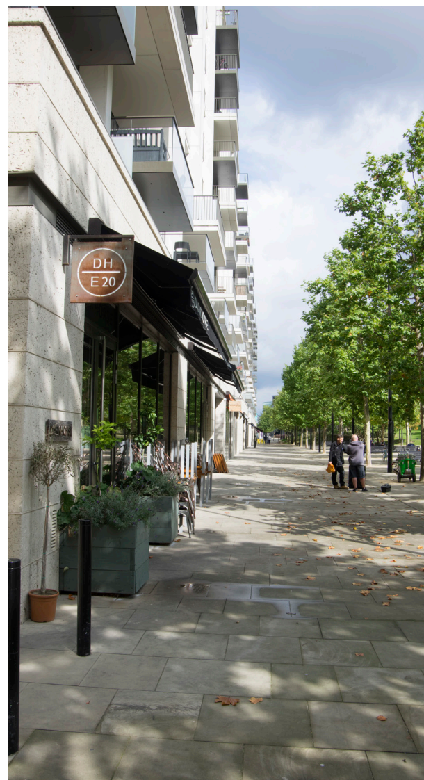
East Village Local Centre
