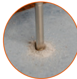
Drilling with slight oscillations. Attention: Please use water for cooling!
