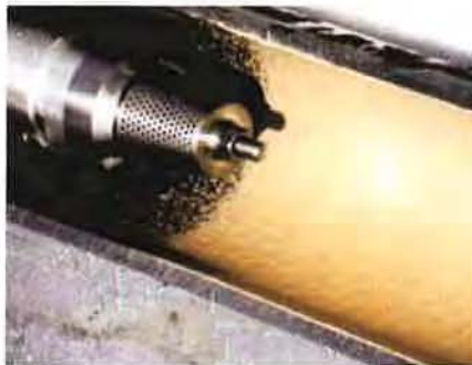
Figure A4-2 Epoxy Lining Spray Head
