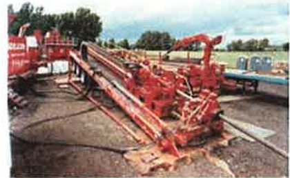
Figure A5-10 Horizontal Drilling Rig
